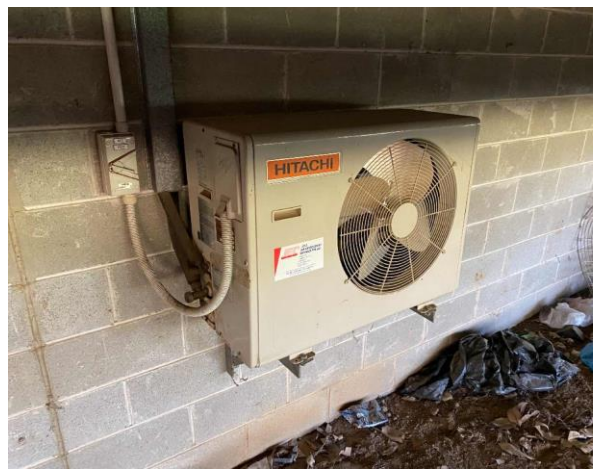
Line ID 40: External, Michael Diamond Building, North Side, Hitachi AC Units, R407C Refrigerant - Non ODS Refrigerant
