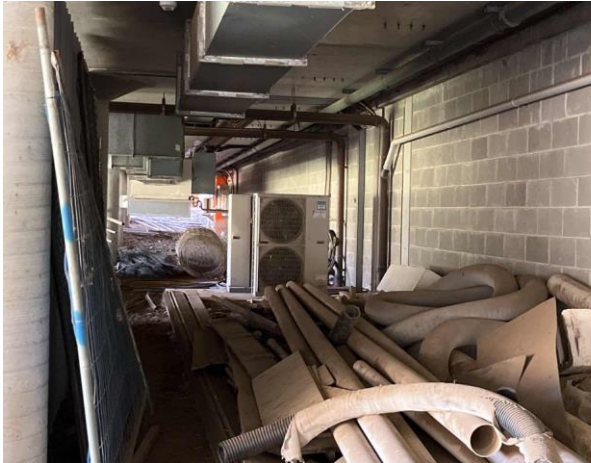
Line ID 41: External, Michael Diamond Building, West Side, Hitachi AC Units, R407C Refrigerant - Non ODS Refrigerant
