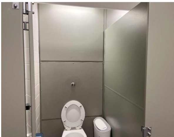
Line ID 11: Internal, Michael Diamond Building, Level 2, Walls Behind Toilets, Fibre Cement Sheet - No Asbestos Detected
