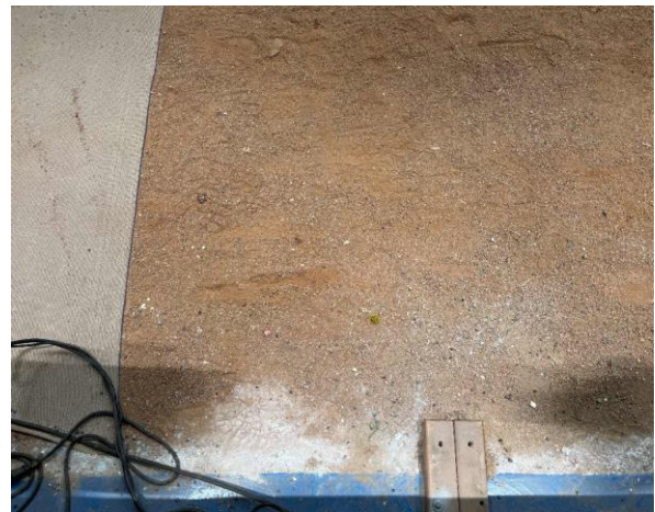
Line ID 28: Internal, Michael Diamond Building, Philip Adams Range 10m Range, Shooting Area, Floor, Dust - Lead Detected (410 mg/kg)
