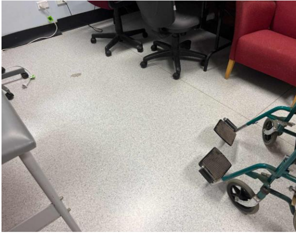
Line ID 13: Internal, Michael Diamond Building, Percy Pavey Range, First Aid Office, Floor Covering, White Vinyl Sheet - No Asbestos Detected
