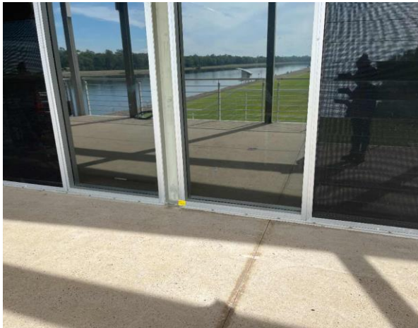
Line ID 12: External, Restaurant, Throughout, Window Frames, Mastic Sealant - No Asbestos Detected
