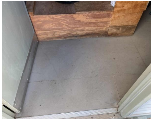
Line ID 53: Internal, Timing Towers, Tower at 0m, Floor Covering, Green Vinyl Sheet - No Asbestos Detected
