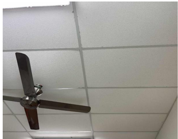
Line ID 92: Internal, Maintenance Shed, Office, Ceiling, Compressed Ceiling Tiles - Suspected SMF
