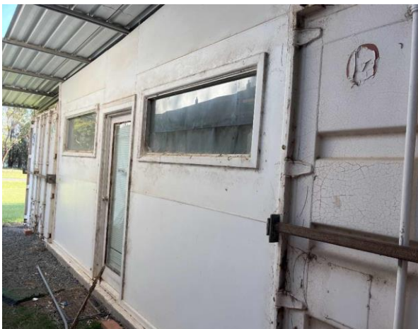
Line ID 10: External, Old Compound, North Building, Wall Between Containers, Fibre Cement Sheet - No Asbestos Detected
