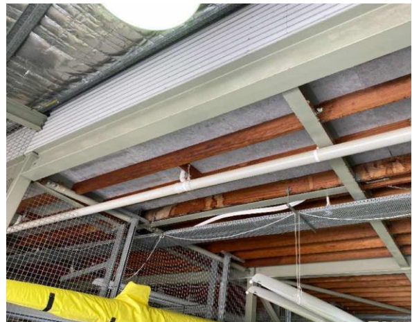
Line ID 20: Internal, Boatsheds, Throughout, Ceiling (Base of Veranda), Compressed Cement Sheeting - No Asbestos Detected
