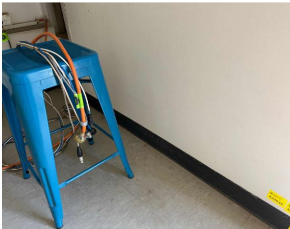
Line ID 50: Internal, Start Line Tower, Throughout, Skirting, Black Vinyl Sheet - No Asbestos Detected
