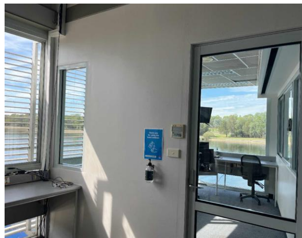
Line ID 33: Internal, Finish Tower, L2, Walls, Fibre Cement Sheet - No Asbestos Detected
