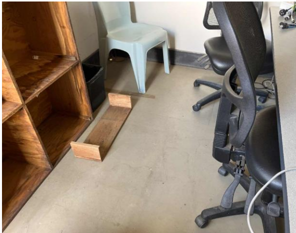
Line ID 64: Internal, Timing Towers, Tower at 1750m, Floor Covering, Green Vinyl Sheet - No Asbestos Detected
