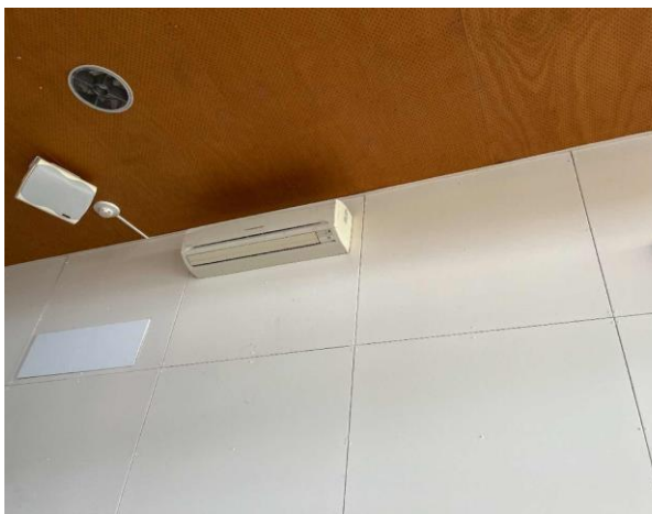
Line ID 116: Internal, Restaurant, East Dining Room, AC Units, Unknown Refrigerant - Suspected ODS
