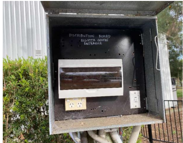
Line ID 15: External, Venue Operations Centre, Throughout, Electrical Pole, Bituminous Backing Board - No Asbestos Suspected
