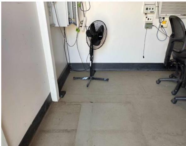
Line ID 60: Internal, Timing Towers, Tower at 1500m, Floor Covering, Green Vinyl Sheet - No Asbestos Detected
