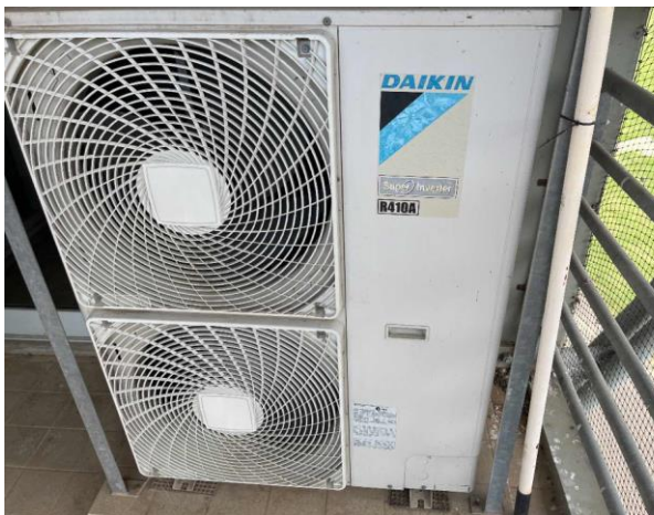
Line ID 105: External, Finish Tower, L2, Balcony, Daikin AC Unit, R410A Hydrofluorocarbon (HFC) - Non ODS Refrigerant
