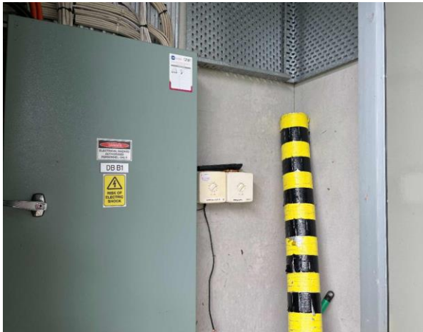
Line ID 1: External, Boatsheds, Meter Rooms, Walls, Fibre Cement Sheeting - No Asbestos Detected
