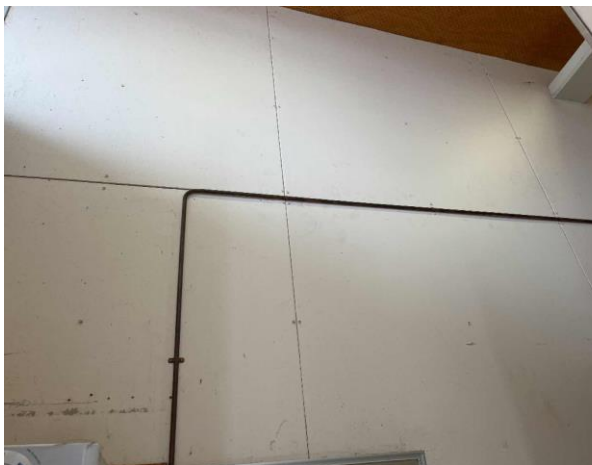
Line ID 44: Internal, Restaurant, North Toilet, Walls, Fibre Cement Sheeting - No Asbestos Detected
