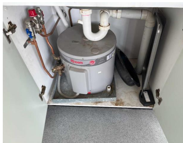
Line ID 88: Internal, Finish Tower, GF, Entrance Hallway, Hot Water Heater, Under Sink, Insulation Material - Suspected SMF
