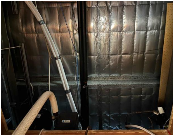
Line ID 95: Internal, Restaurant, Kitchen, Ceiling Space, Sarking Insulation - Suspected SMF
