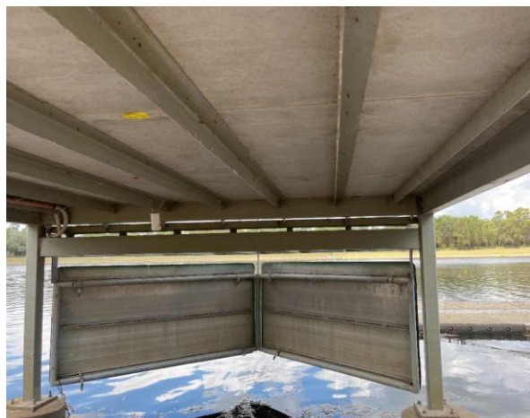
Line ID 57: Internal, Timing Towers, Tower at 1000m, Floor Lining below Vinyl, Fibre Cement Sheet - No Asbestos Detected
