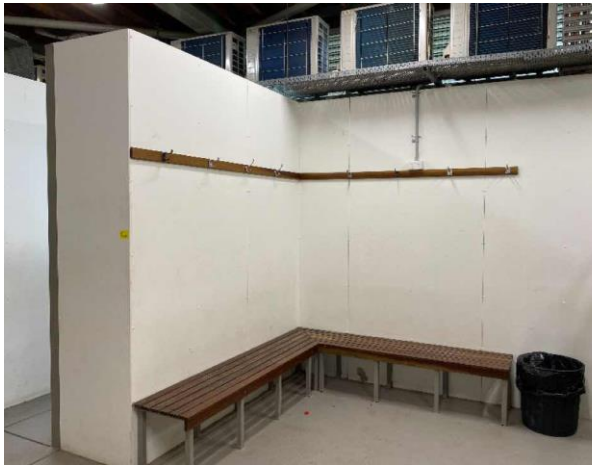
Line ID 17: Internal, Boatsheds, Female Toilets, Walls, Fibre Cement Sheeting - No Asbestos Detected
