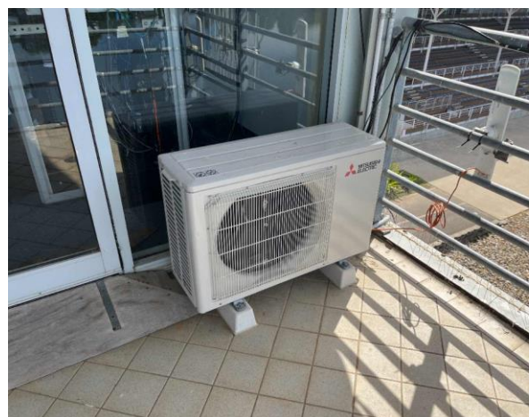
Line ID 107: External, Finish Tower, L3, Balcony, Mitsubishi AC Unit, R32 Refrigerant - Non ODS Refrigerant
