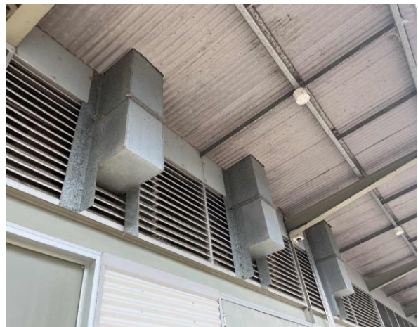
Line ID 11: External, Restaurant, Throughout, Fascia, Fibre Cement Sheet - No Asbestos Detected
