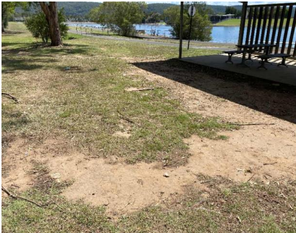
Line ID 8: External, Grounds, South East Picnic Area, Ground Surface, Debris - Chrysotile, Amosite and Crocidolite Asbestos Detected
