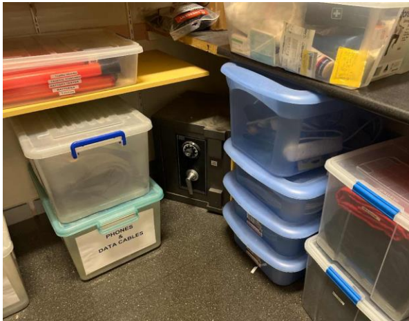
Line ID 58: Internal, Venue Office, Office A.05, Safe, Internal Insulation - Suspected Asbestos
