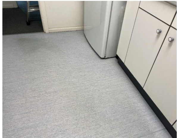
Line ID 30: Internal, House, Kitchen, Floor Covering, Blue Vinyl Sheet - No Asbestos Detected
