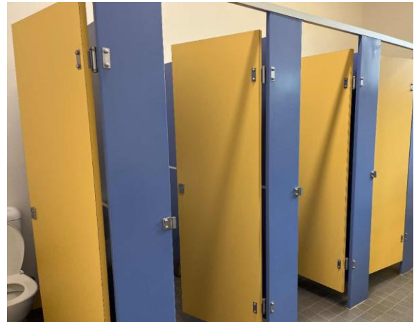
Line ID 59: Internal, Venue Office, Toilets, Cubicle Walls, Compressed Cement Sheeting - No Asbestos Detected
