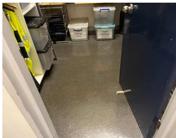
Line ID 57: Internal, Venue Office, Office A.05, Floor Covering, Grey Vinyl Sheet - No Asbestos Detected
