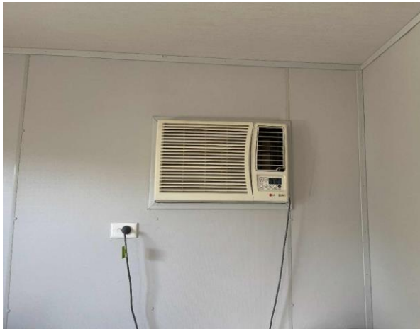
Line ID 93: Internal, Riders Retreat, First Aid Room, LG AC Unit, Unknown Refrigerant - Suspected ODS
