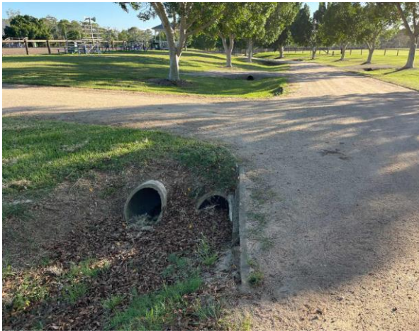
Line ID 3: External, Grounds Throughout, East of Arena 2, Drainage Pipes, Moulded Fibre Cement - No Asbestos Detected
