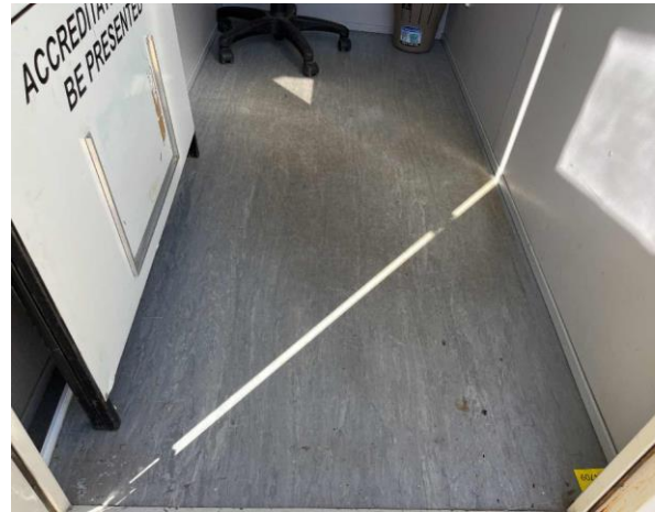
Line ID 48: Internal, Security Hunts on Road, Throughout, Floor Covering, Grey Vinyl Sheet - No Asbestos Detected
