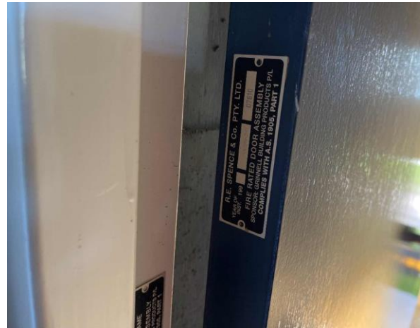
Line ID 36: Internal, Main Arena 1, Western Storage Area, Door to F.06, F.03 and F.05, Fire Door Core - Suspected Asbestos
