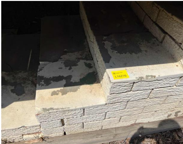
Line ID 64.1: External, House, Perimeter, Walls and Old Stairs, Cream Paint - Lead Detected (<0.005% w/w)
