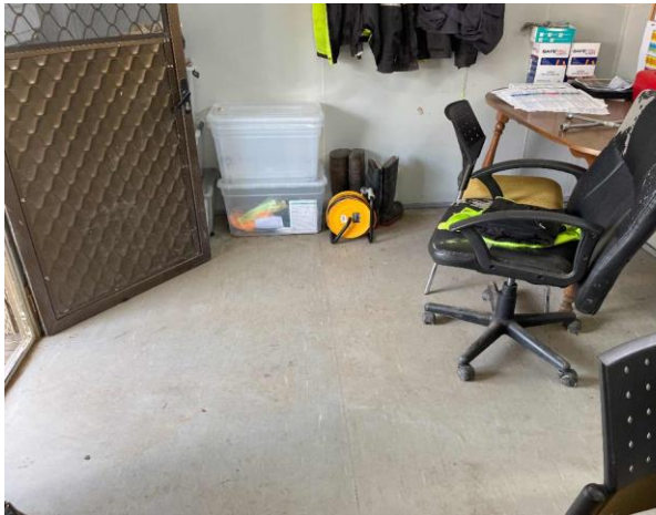
Line ID 23: Internal, Gardener's Shed, Lunch Shed, Floor Covering, Blue Vinyl Sheet - No Asbestos Detected
