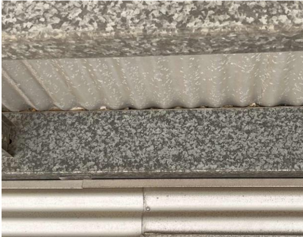
Line ID 72: Internal, Indoor Arena, Judges Office, Ceiling Void, Insulation Material - Suspected SMF
