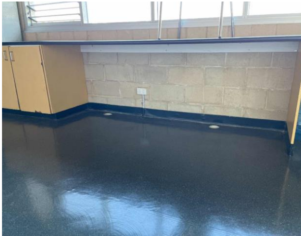
Line ID 35: Internal, Main Arena 1, Eastern Storage Area, E.03 Skirting, Black Vinyl Sheet - No Asbestos Detected
