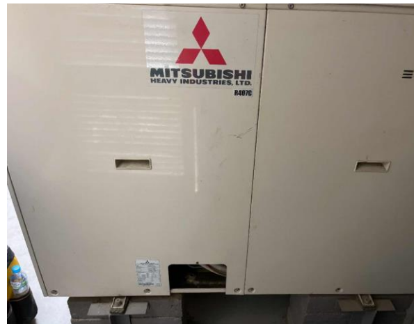
Line ID 96: Internal, Venue Office, Electrical Comms A.15, Mitsubishi AC Unit, R407c Refrigerant - Non ODS Refrigerant
