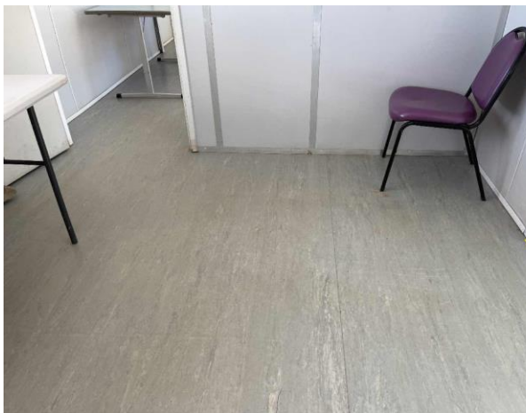
Line ID 45: Internal, Riders Retreat, Event Office, Floor Covering, Blue Vinyl Sheet - No Asbestos Detected
