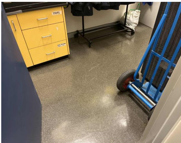
Line ID 55: Internal, Venue Office, Office A.02, Floor Covering, Grey Vinyl Sheet - No Asbestos Detected
