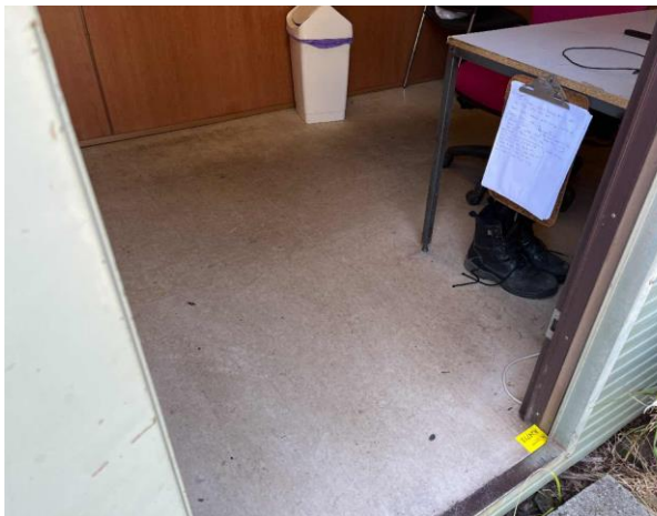
Line ID 49: Internal, Security Office, Throughout, Floor Covering, Grey Vinyl Sheet - No Asbestos Detected
