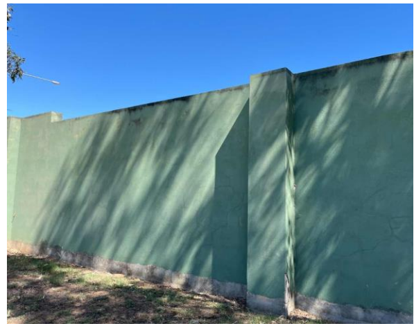
Line ID 61: External, Grounds Throughout, Perimeter, North and West Walls, Green Paint - Lead Detected (<0.005% w/w)
