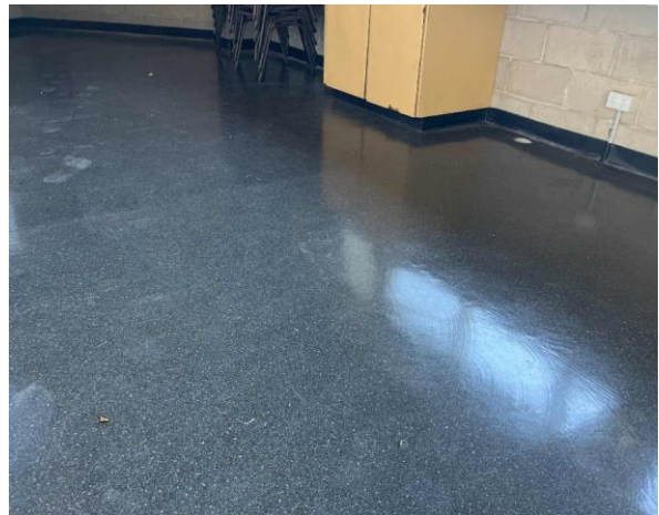
Line ID 33: Internal, Main Arena 1, Eastern Storage Area, E.03 Floor Covering, Black Vinyl Sheet - No Asbestos Detected
