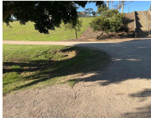
Line ID 3.1: External, Grounds Throughout, East of Arena 2, Drainage Pipes, Moulded Fibre Cement - No Asbestos Detected
