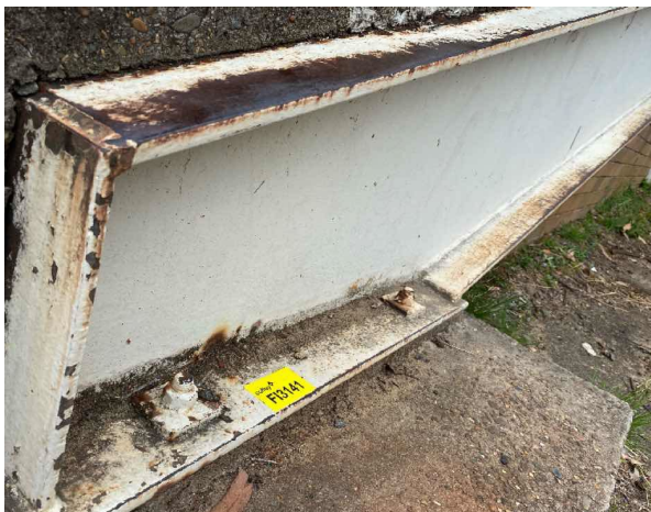
Line ID 48: External, Athletics Track Stand, Seating Area, Metal Beams, Cream Paint - Lead Detected (0.008% w/w)
