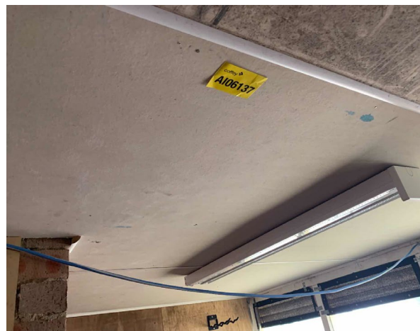
Line ID 36: Internal, Gymnasium, Cleaners Rooms, Ceiling Lining, Fibre Cement Sheet - No Asbestos Detected
