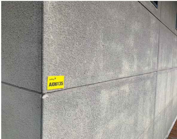
Line ID 13: External, Oval 3 Toilet Block and Change Rooms, Elevations, Facia Panels, Compressed Cement Sheet - No Asbestos Detected
