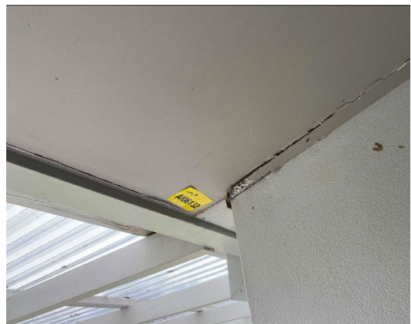
Line ID 18: External, Rugby Field Office, Perimeter, Eaves, Compressed Cement Sheet - No Asbestos Detected
