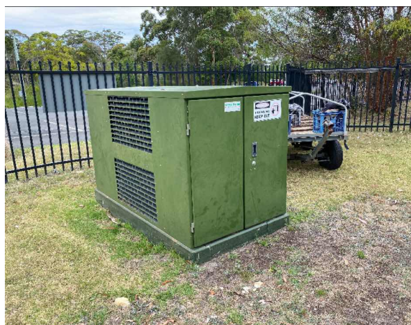
Line ID 87: External, Athletics Track Stand, Adjacent Toilet Side Entry Gate, Green Transformer, Ballast(s) - Suspected PCB
