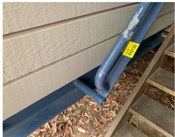
Line ID 51: External, Dorm Accommodation 1-12, Elevations, Metal, Support Structures, Trimwork and Handrails, Blue Paint - Lead Detected (0.01% w/w)
