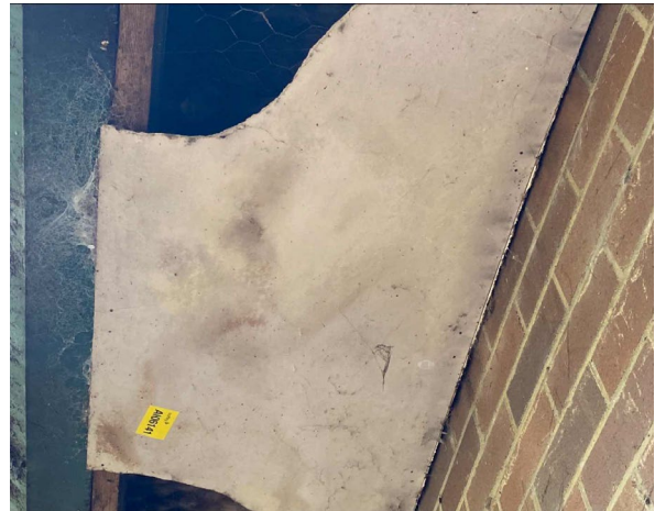
Line ID 16: External, Pump House, Elevations, Eaves, Compressed Cement Sheet - No Asbestos Detected
