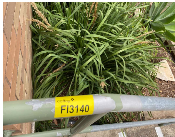
Line ID 49: External, Athletics Track Stand, Toilet Block, Adjacent Entry, Handrail, Green (Light) Paint - Lead Detected (0.005% w/w)
