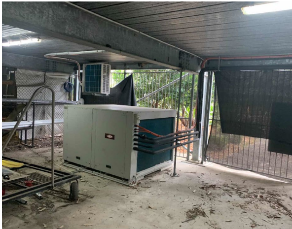
Line ID 88: External, Administration Office, Basement Carpark, Air Conditioning Unit, R22 Hydrochlorofluorocarbon (HCFC) - ODS Refrigerant
