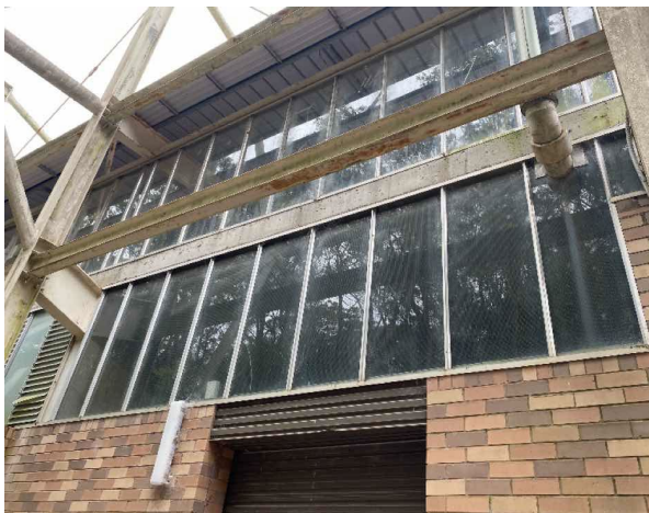
Line ID 3: External, Athletics Track Stand, Seating Area, Rear Adjacent Access Gate, Pipework, Moulded Fibre Cement - Suspected Asbestos
