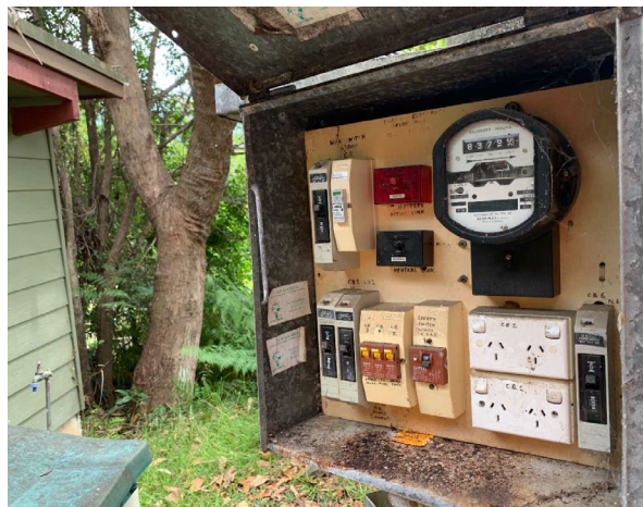
Line ID 26: External, Staff Residence #1 (South of Dining Dorm), North Side of House, Electrical Switchboard, Bituminous Backing Board - Chrysotile Asbestos Detected
