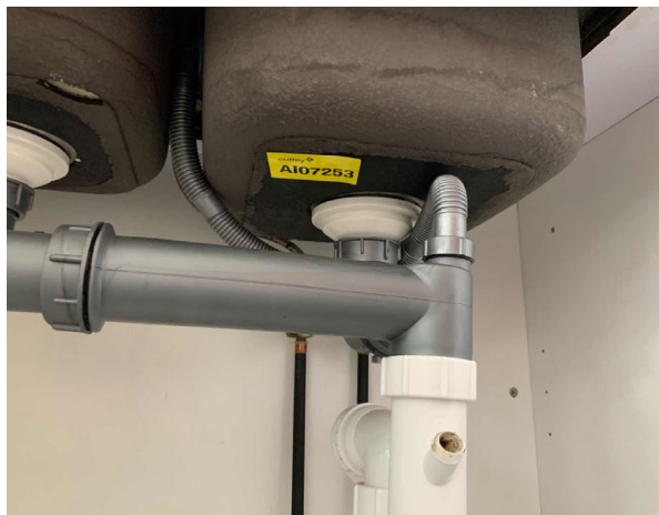
Line ID 40: Internal, Sea Eagles Coaching Offices, Kitchenette, Beneath Sink, Bituminous Sink Pad - No Asbestos Detected
