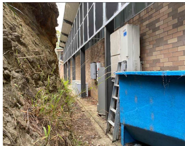
Line ID 68: External, Athletics Track Stand, South Wall, Hot Water Heater, Internal Insulation - Suspected SMF
