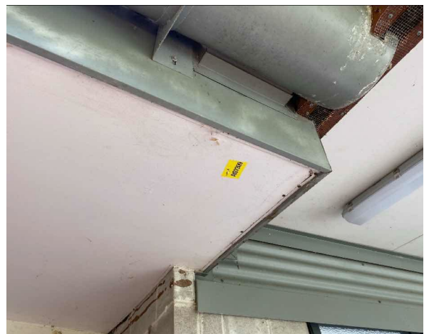
Line ID 6: External, Dining Dorm, Perimeter, Eaves, Fibre Cement Sheet - No Asbestos Detected
