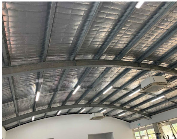
Line ID 85: Internal, Weights Room, Throughout, Underside of Roof, Sarking Insulation - Suspected SMF
