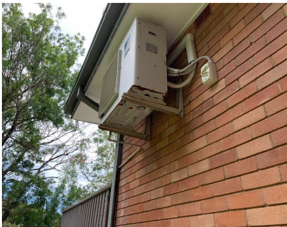
Line ID 62: External, Staff Residence #3 (West of Dining Dorm), Building Perimeter, Eaves, White Paint - Lead Detected (0.2% w/w)
