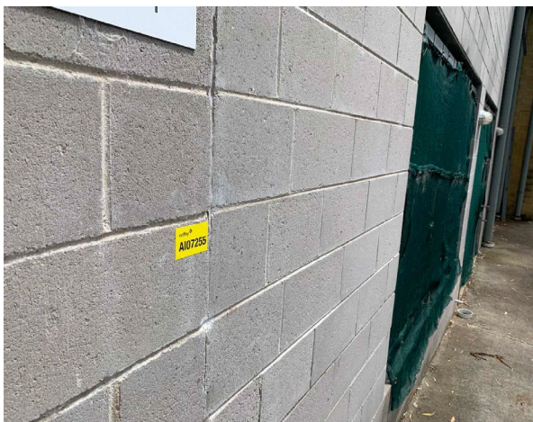
Line ID 5: External, Dining Dorm, Perimeter, Concrete Block Work, Vertical Joints Throughout, Construction Joint Mastic - Chrysotile Asbestos Detected
