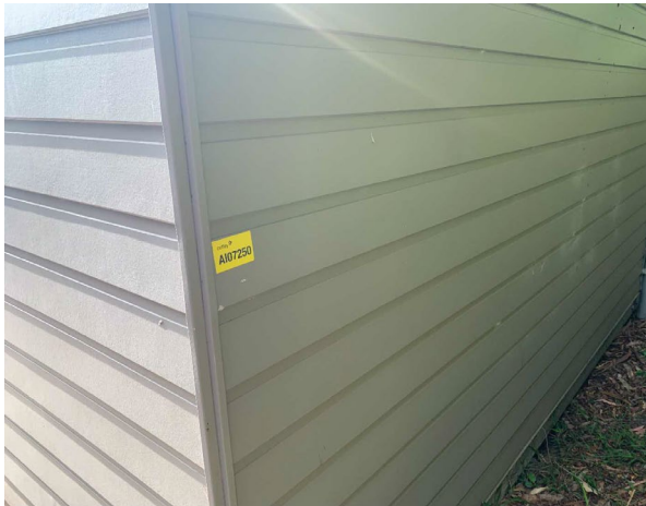
Line ID 9: External, Dorm Accommodation 1-12, Elevations, North and Northeast Fascia, Panelling, Compressed Cement Sheet - No Asbestos Detected
