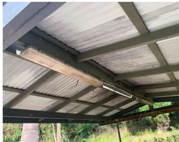
Line ID 64: External, The Compound, Gardeners Shed, Timber Framework, Brown Paint - Lead Detected (0.3% w/w)
