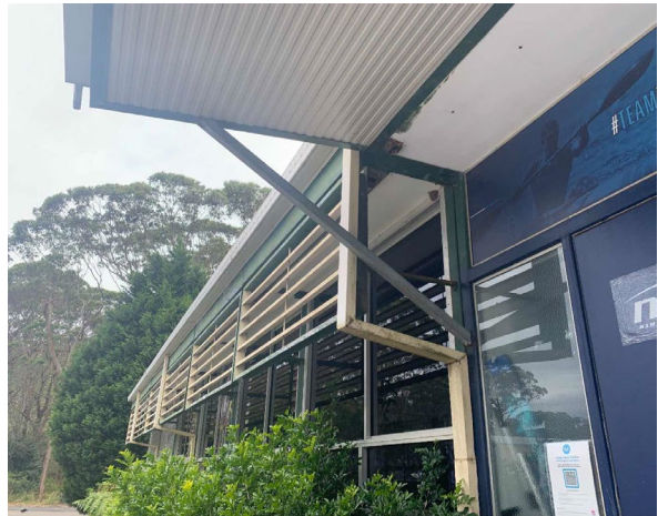
Line ID 20: External, Sea Eagles, North Side Demountable, Entrance Ceiling Lining, Fibre Cement Sheet - Chrysotile Asbestos Detected
