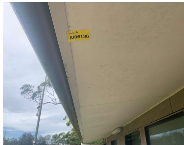
Line ID 12: External, Oval 3 Toilet Block and Change Rooms, Elevations, Eaves, Fibre Cement Sheetting - No Asbestos Detected
