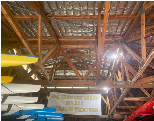
Line ID 75: Internal, Boat Shed, Throughout, Underside of Roof, Sarking Insulation - Suspected SMF
