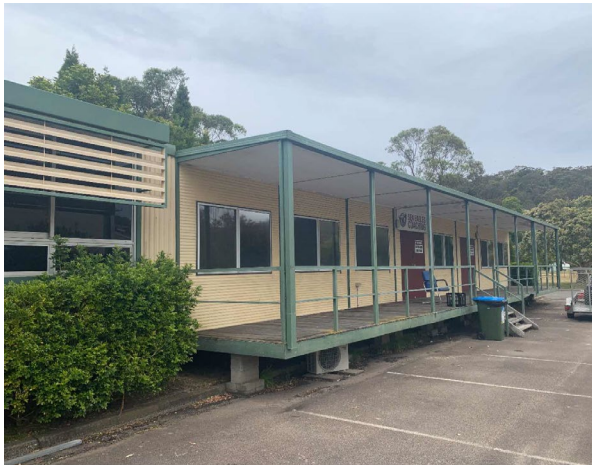
Line ID 21: External, Sea Eagles, North Side Demountable, Entrance Eaves Lining, Fibre Cement Sheet - Chrysotile Asbestos Detected
