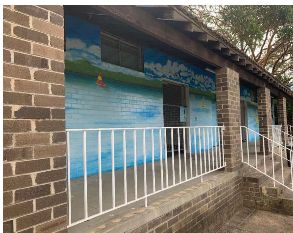
Line ID 55: External, Picnic Toilet Block, Framework, Throughout, White Paint - Lead Detected (0.3% w/w)
