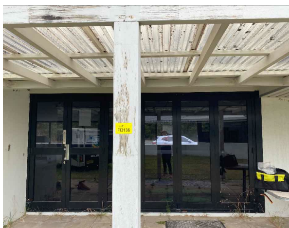
Line ID 56: External, Rugby Field Office, Perimeter, Timberwork, White Paint - Lead Detected (<0.005% w/w)
