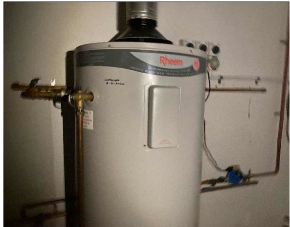
Line ID 72: Internal, Aquatics Facility, Plant Room, Rheem Hot Water Unit, Internal Insulation - Suspected SMF
