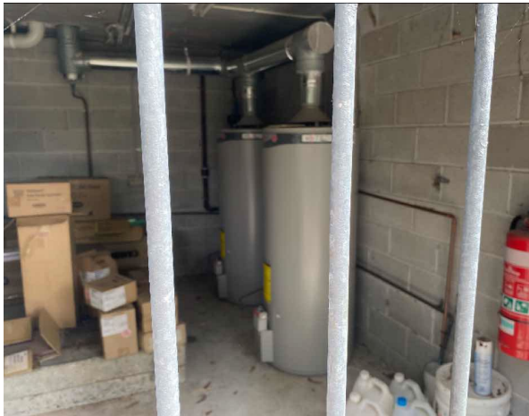
Line ID 69: External, Dining Dorm, Plant Rooms Adjacent Car Park, Hot Water Heater, Internal Insulation - Suspected SMF
