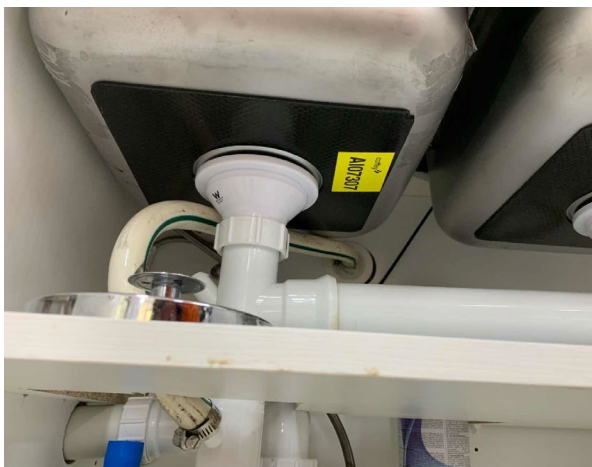
Line ID 35: Internal, Dining Dorm, Level 1, Kitchenette, Beneath Sink, Bituminous Sink Pad - No Asbestos Detected
