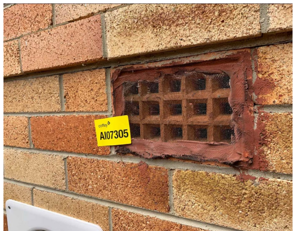
Line ID 24: External, Staff Residence #1 (South of Dining Dorm), Building Perimeter, Ventilation Grate, Mastic Sealant, Mastic Sealant - No Asbestos Detected
