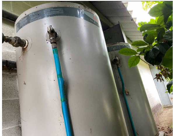
Line ID 70: External, Sea Eagles, Gym West Face, Hot Water Units, Internal Insulation - Suspected SMF
