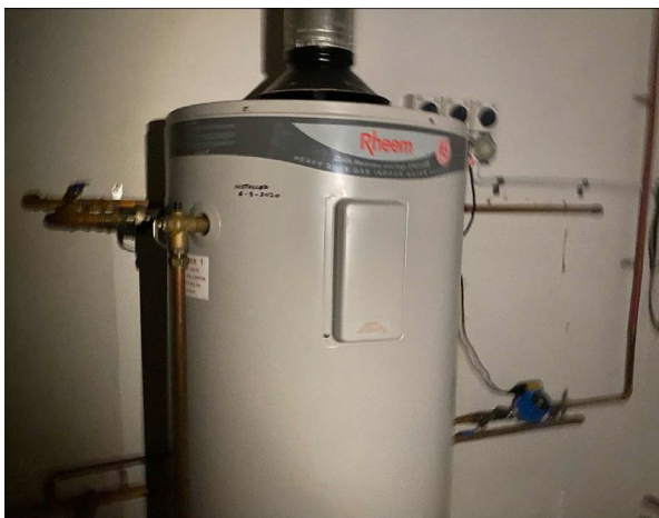
Line ID 79: Internal, Lecture Rooms and Motel Accommodation, Cleaners Storage Room, Hot Water Heater, Internal Insulation - Suspected SMF
