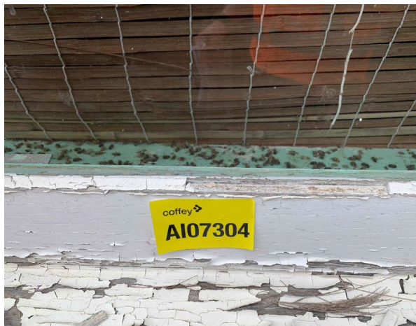
Line ID 25: External, Staff Residence #1 (South of Dining Dorm), Building Perimeter, Window Frames, Pane to Timber Joint, Window Caulking - No Asbestos Detected
