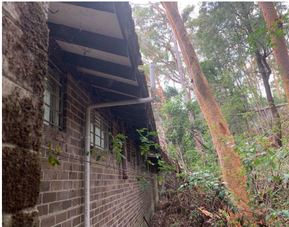
Line ID 15: External, Picnic Toilet Block, Rear, Eaves Lining, Fibre Cement Sheet - Chrysotile Asbestos Detected
