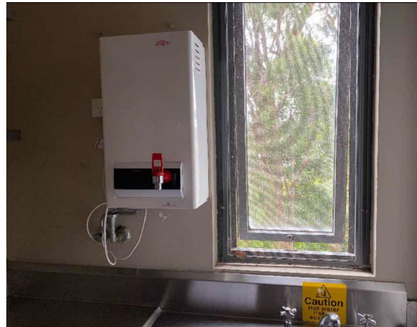
Line ID 76: Internal, Dining Dorm, Wash Area, Hot Water Heater, Internal Insulation - Suspected SMF
