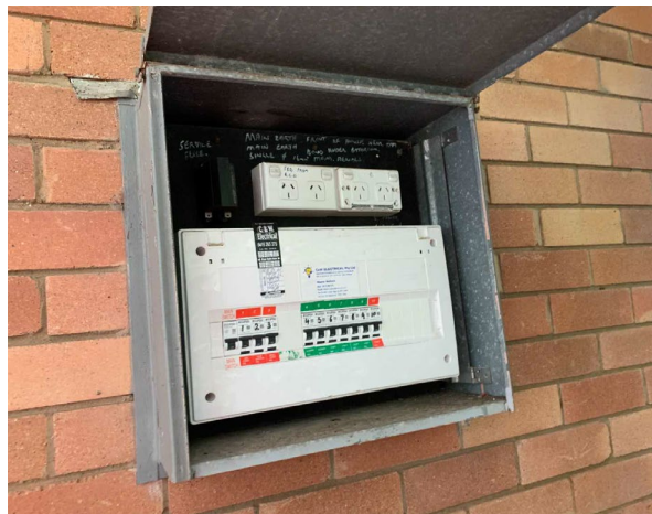
Line ID 28: External, Staff Residence #3 (West of Dining Dorm), Carport, Front of House, Electrical Switchboard, Bituminous Backing Board - Chrysotile Asbestos Detected
