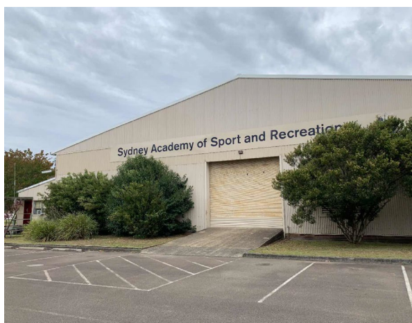
Line ID 52: External, Gymnasium, Building Perimeter, Guttering, Green Paint - Lead Detected (0.2% w/w)
