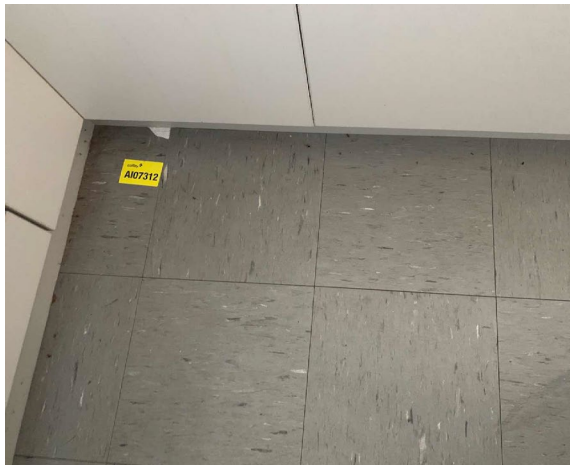
Line ID 33: Internal, Bilgola House, Kitchen and Wet Areas, Floor Covering, Grey Vinyl Floor Tiles - No Asbestos Detected
