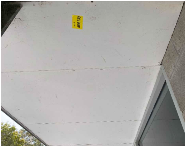
Line ID 19: External, Sea Eagles, Gym Perimeter, Eaves, Fibre Cement Sheet - No Asbestos Detected
