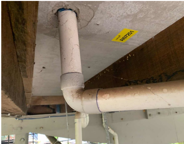
Line ID 7: External, Dorm Accommodation 1-12, Building Perimeter , All Units, Subfloor, Beneath Wet Areas, Compressed Cement Sheet - No Asbestos Detected
