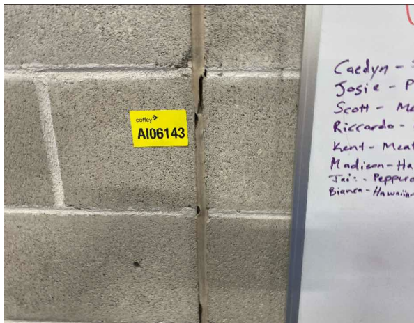
Line ID 38: Internal, Gymnastics, Training Area, Perimeter Walls, Construction Joint Mastic - No Asbestos Detected
