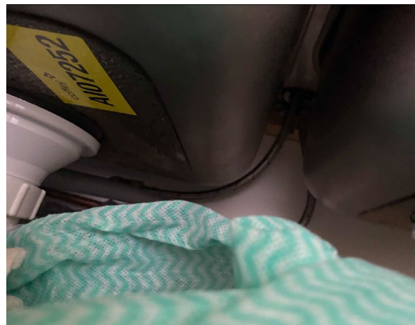
Line ID 41: Internal, Staff Accommodation (Five Domiciles), Kitchen and Wet Areas, Kitchen, Beneath Sink, Bituminous Sink Pad - No Asbestos Detected
