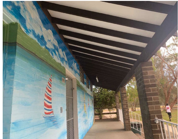
Line ID 14: External, Picnic Toilet Block, Entrance Awning, Lining, Fibre Cement Sheet - Chrysotile Asbestos Detected
