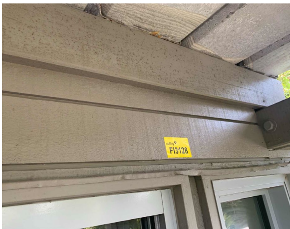
Line ID 65: Internal, Dorm Accommodation 1-12 (Former Staff Accom), Throughout, All Dorms, Fascia, Dark Green/Grey Paint - Lead Detected (0.02% w/w)
