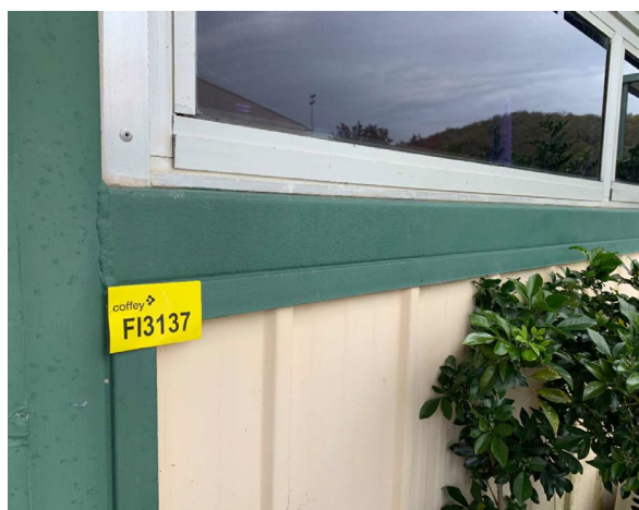
Line ID 57: External, Sea Eagles Coaching, Elevations, Trimwork, Green Paint - Lead Detected (0.084% w/w)
