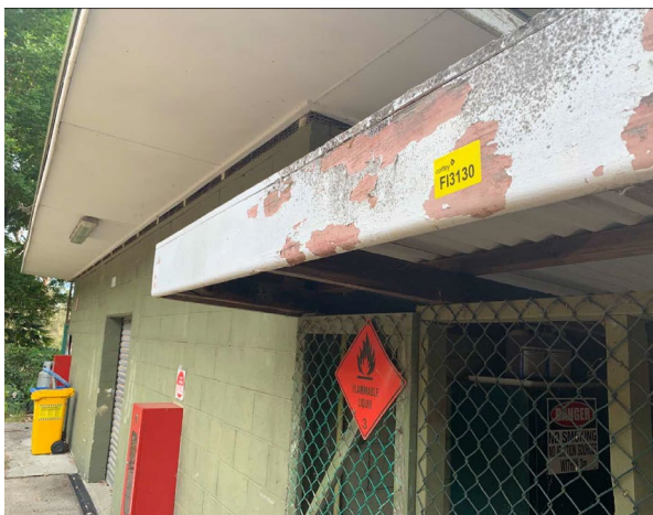
Line ID 50: External, Chemical Shed, Throughout, Trimwork, White Paint - Lead Detected (0.12% w/w)
