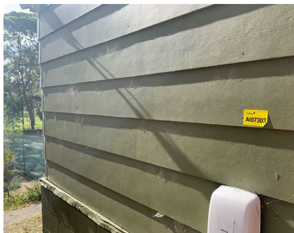
Line ID 30: External, Tennis Court Building, Perimeter, Facia Panelling, Compressed Cement Sheet - No Asbestos Detected
