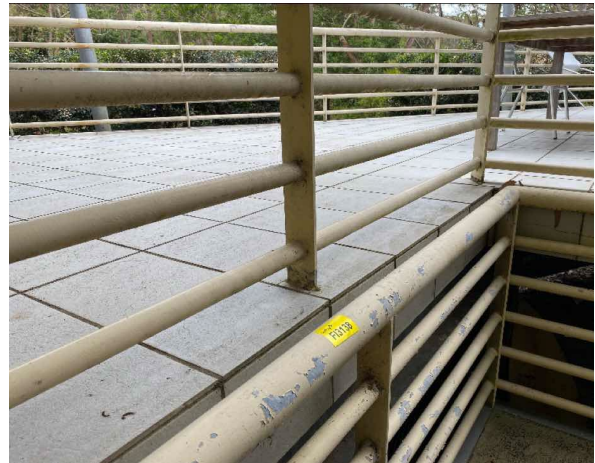
Line ID 47: External, Administration Office, Perimeter, Handrails Throughout, Cream Paint - Lead Detected (0.01% w/w)
