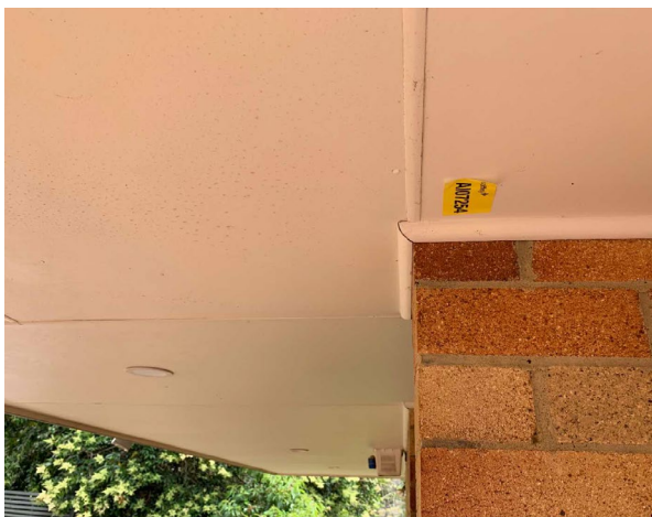
Line ID 23: External, Staff Residence #1 (South of Dining Dorm), Building Perimeter, Eaves and Awnings, Fibre Cement Sheet - No Asbestos Detected
