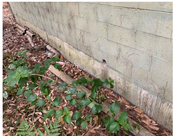
Line ID 4: External, Chemical Shed, Rear, Ground, Redundant Pipe, Moulded Cement Pipe - Chrysotile, Amosite and Crocidolite Asbestos Detected
