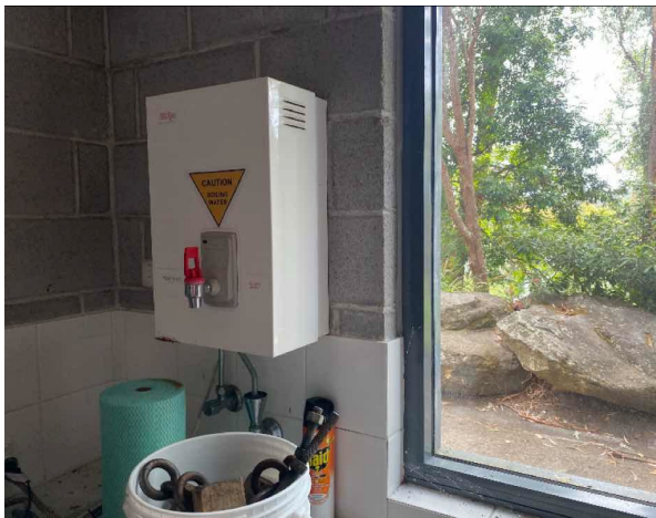
Line ID 77: Internal, Dining Dorm, Storeroom, Boiler, Internal Insulation - Suspected SMF
