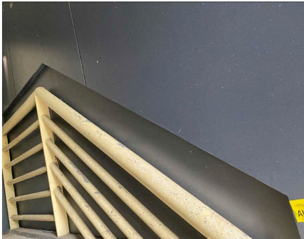
Line ID 1: External, Administration Office, Perimeter, Upper Perimeter Walls, Compressed Cement Sheet - No Asbestos Detected
