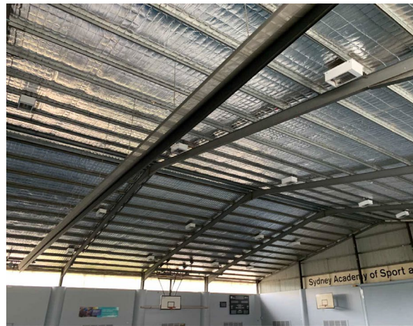
Line ID 78: Internal, Gymnasium, Basketball Court, Roof Lining, Sarking Insulation - Suspected SMF
