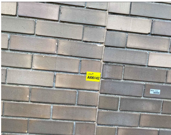
Line ID 11: External, Motel Accommodation, Elevations, Walls, Vertical Joints Throughout, Construction Joint Mastic - No Asbestos Detected
