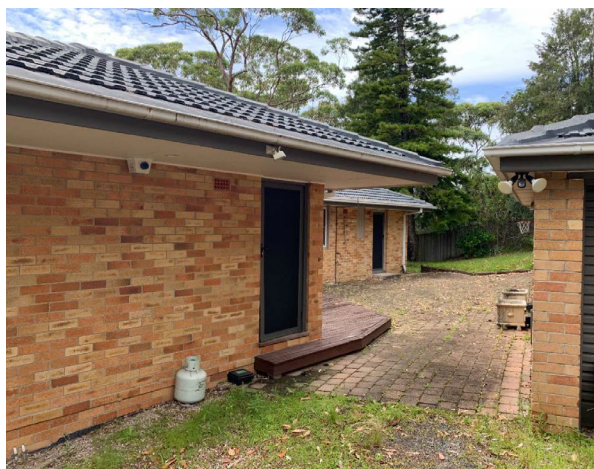
Line ID 29: External, Staff Residence 3 (West of Picnic Area), Building Perimeter, Eaves, Fibre Cement Sheet - Chrysotile Asbestos Detected
