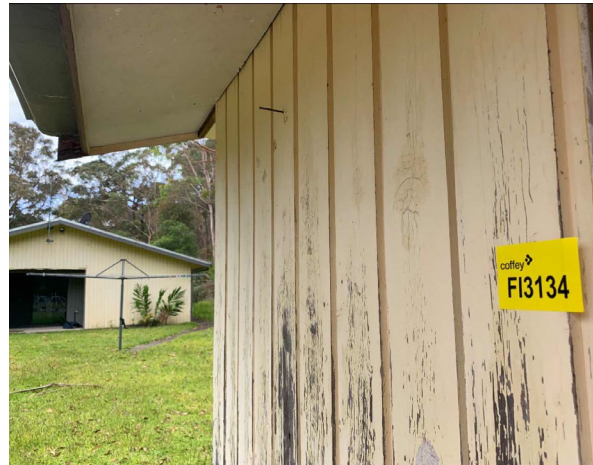
Line ID 61: External, Staff Residence #2 (West of Dining Room), Shed, Throughout, Yellow (Light) Paint - Lead Detected (<0.005% w/w)
