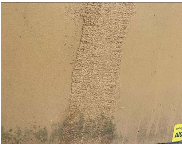
Line ID 17: External, Pump House, Elevations, Yellow Wall Panelling, Compressed Cement Sheet - No Asbestos Detected
