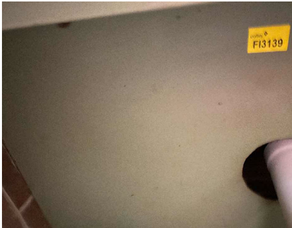
Line ID 46: Internal, Weights Room, Switch Cupboard, Ceiling, Fibre Cement Sheet - No Asbestos Detected
