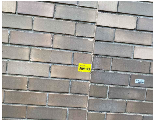
Line ID 10: External, Lecture Rooms and Accommodation, Deliveries Entrance, Brick Wall Adjacent Door, Construction Joint Mastic - No Asbestos Detected
