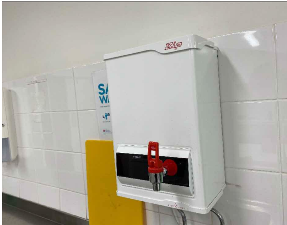
Line ID 71: Internal, Administration Building, Kitchen, Zip Hot Water Unit, Internal Insulation - Suspected SMF
