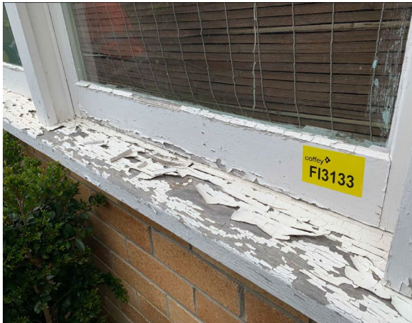
Line ID 60: External, Staff Residence #1 (South of Dining Dorm), Building Perimeter, Window Frames and Trimwork, White Paint - Lead Detected (0.72% w/w)
