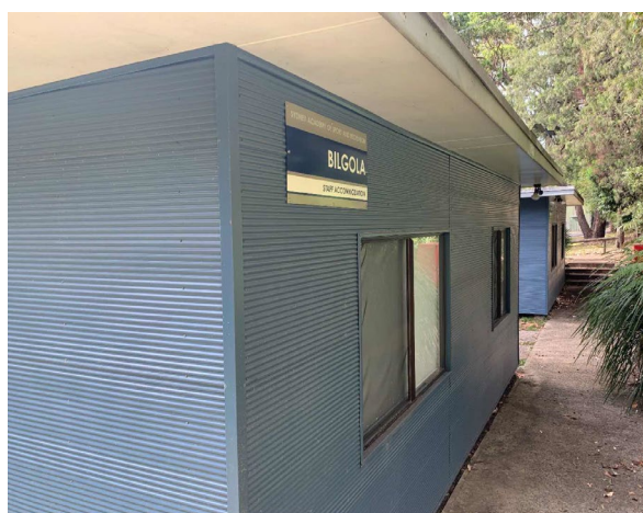
Line ID 59: External, Staff Accommodations (Five Domiciles), Elevations, Eaves, White Paint - Lead Detected (0.41% w/w)
