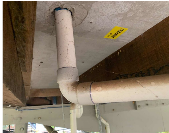
Line ID 8: External, Dorm Accommodation 1-12, Building Perimeter , Freshwater 1, Subfloor, Below Wet Areas, Compressed Cement Sheet - No Asbestos Detected
