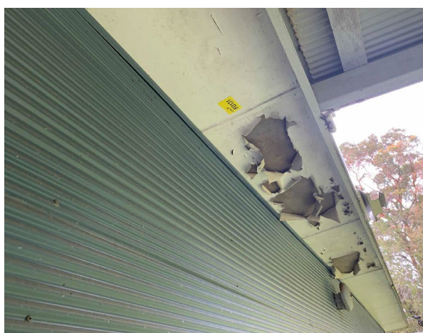
Line ID 58: External, Staff Accommodations (Five Domiciles), Elevations, Bilgoa, Eaves, White Paint - Lead Detected (0.41% w/w)
