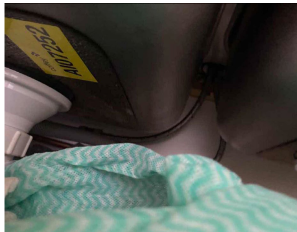
Line ID 39: Internal, Rooms Adjacent East Picnic Area, Kitchen, Beneath Sink, Bituminous Sink Pad - No Asbestos Detected
