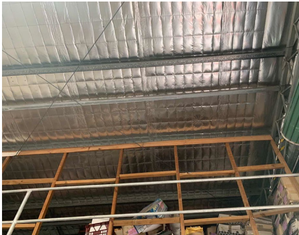
Line ID 81: Internal, Mower Room, Throughout, Underside of Roof, Sarking Insulation - Suspected SMF
