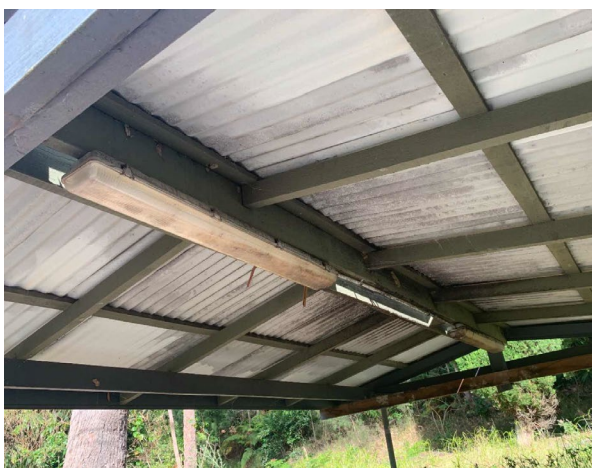
Line ID 86: Internal, Workshop, Throughout, Underside of Roof, Sarking Insulation - Suspected SMF
