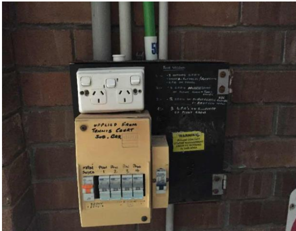
Line ID 79: Internal, GF, Pool House, Pool Store & Toilet Block, Western Wall of Pump House, Bituminous Backing Board - Suspected Asbestos
