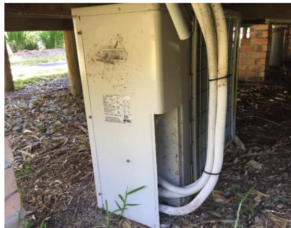
Line ID 156: External, GF, Conference Lodge, Beneath Building, Air Conditioning Unit, R410A Hydrofluorocarbon (HFC) - Non ODS Refrigerant
