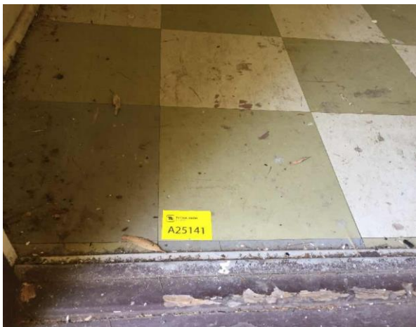
Line ID 63: Internal, GF, Bush Craft Building, Eastern and Southern Rooms, Olive Green Vinyl Floor Tiles - Chrysotile Asbestos Detected
