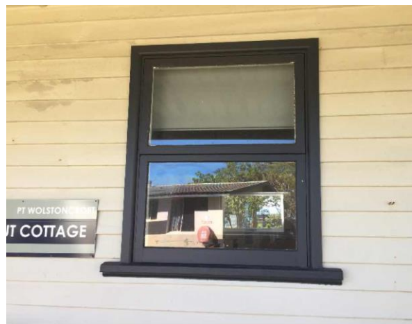
Line ID 101: External, GF, Gum Nut Lodge, Door, Window Frames and Trim, Grey (Dark) Paint - Lead Detected (1.9% w/w)
