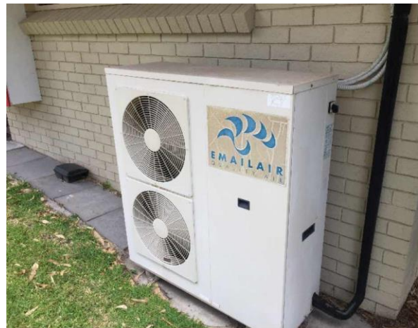
Line ID 154: External, GF, Administration/Office Building, Southern Elevation, Air Conditioning Unit, R22 Hydrochlorofluorocarbon (HCFC) - ODS Refrigerant
