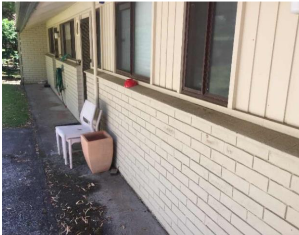
Line ID 108: External, GF, Residence 2 (Wattle House & Garage), House and Garage Walls, Beige Paint - Lead Detected (0.005% w/w)
