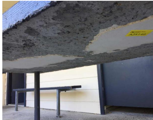
Line ID 50: External, GF, Tennis Court Amenities Block (North), Underside of Concrete Table, Fibre Cement Sheetting - Chrysotile Asbestos Detected
