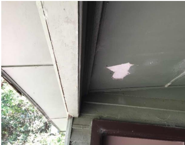
Line ID 9: External, GF, Bush Craft Building, Eaves and Porch Ceiling, Fibre Cement Sheetting - Chrysotile & Amosite Asbestos Detected
