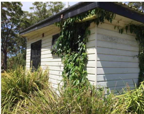
Line ID 112: External, GF, Ropes Course Store Building/Toilet, Walls, Beige Paint - Lead Detected (<0.005% w/w)
