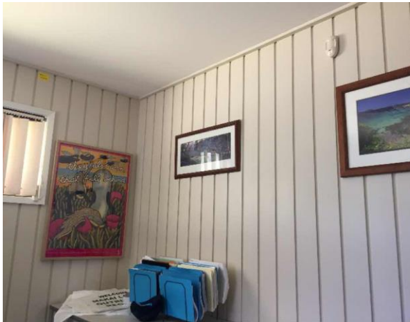
Line ID 114: Internal, GF, Administration/Office Building, Walls Throughout, Cream Paint - Lead Detected (0.02% w/w)
