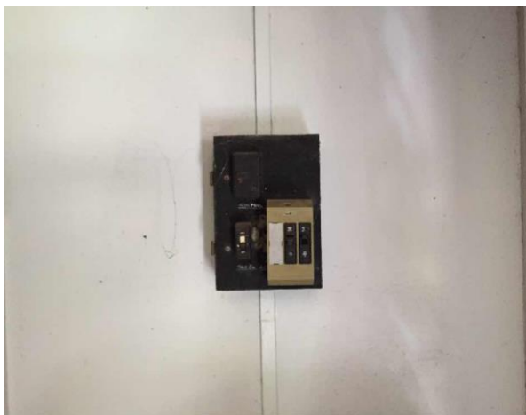
Line ID 71: Internal, GF, Equipment Store Building, West Wall, Bituminous Backing Board - Chrysotile Asbestos Detected
