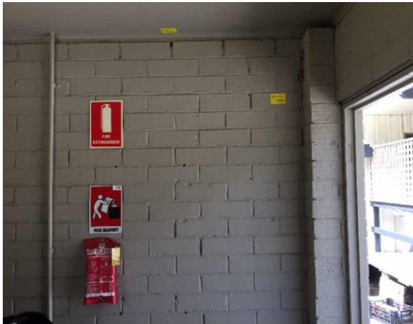
Line ID 120: Internal, GF, Holiday Units (1-8) Laundry, Walls and Ceiling, Grey Paint - Lead Detected (0.02% w/w)
