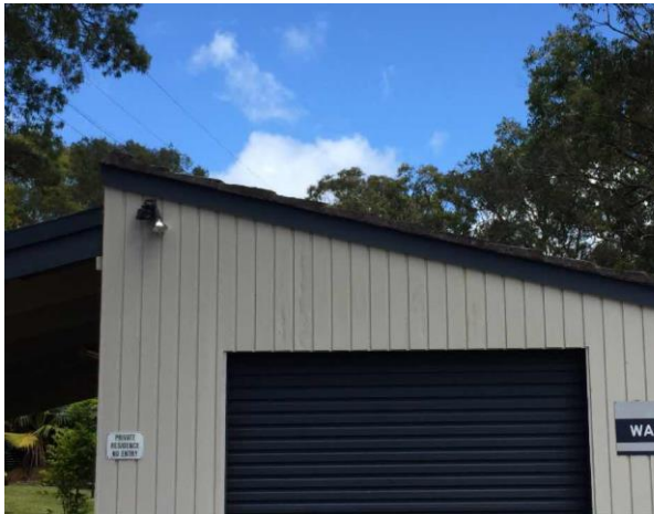
Line ID 33: External, GF, Residence 1 (Waratah House & Garage), Garage, Under Roof Tiles, Compressed Cement Sheeting - Chrysotile Asbestos Detected
