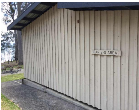
Line ID 94: External, GF, Barbeque Area, Walls Throughout, Beige Paint - Lead Detected (<0.005% w/w)
