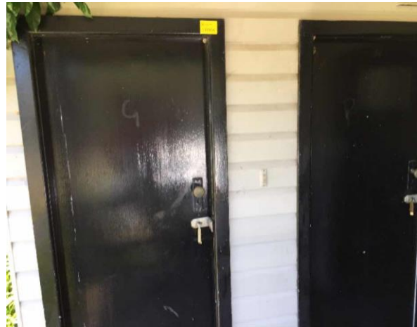
Line ID 111: External, GF, Ropes Course Store Building/Toilet, Hand-railing, Doors, Window and Door Frames, Black Paint - Lead Detected (0.20% w/w)
