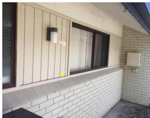
Line ID 107: External, GF, Residence 1 (Waratah House & Garage), House and Garage Walls, Beige Paint - Lead Detected (0.005% w/w)
