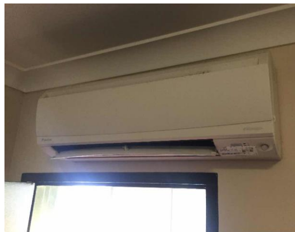
Line ID 168: Internal, GF, Geebung Lodge, Air Conditioning Units, R410A Hydrofluorocarbon (HFC) - Non ODS Refrigerant
