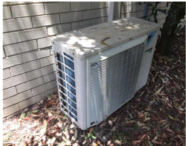
Line ID 162: External, GF, Residence 1 (Waratah House & Garage), Eastern Wall, Air Conditioning Unit, R32 Refrigerant - Non ODS Refrigerant
