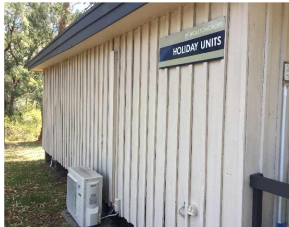
Line ID 105: External, GF, Holiday Units 1-8 (All Identical In Design), Walls Throughout, Beige Paint - Lead Detected (<0.005% w/w)
