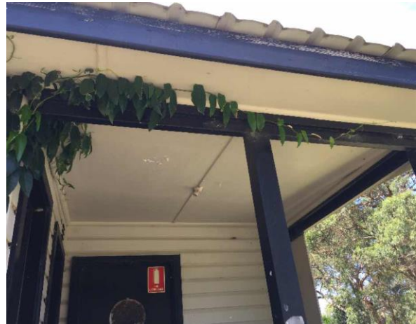
Line ID 44: External, GF, Ropes Course Store Building/Toilet, Eaves and Porch Ceiling, Fibre Cement Sheeting - Chrysotile & Amosite Asbestos Detected
