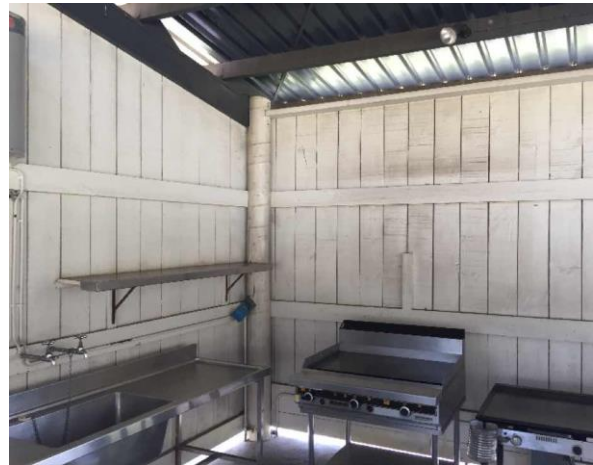
Line ID 115: Internal, GF, Barbeque Area, Walls Throughout, Beige Paint - Lead Detected (<0.005% w/w)
