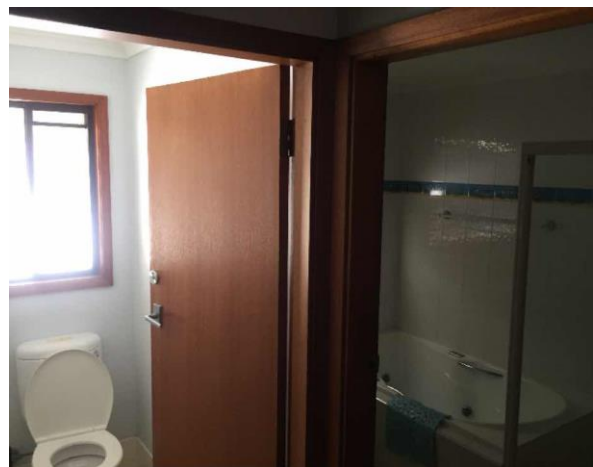
Line ID 83: Internal, GF, Residence 2 (Wattle House & Garage), Laundry, Toilet and Bathroom Walls, Fibre Cement Sheetting - Chrysotile Asbestos Detected
