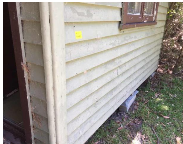
Line ID 95: External, GF, Bush Craft Building, Walls and Eaves, Green Paint - Lead Detected (0.15mg/kg)
