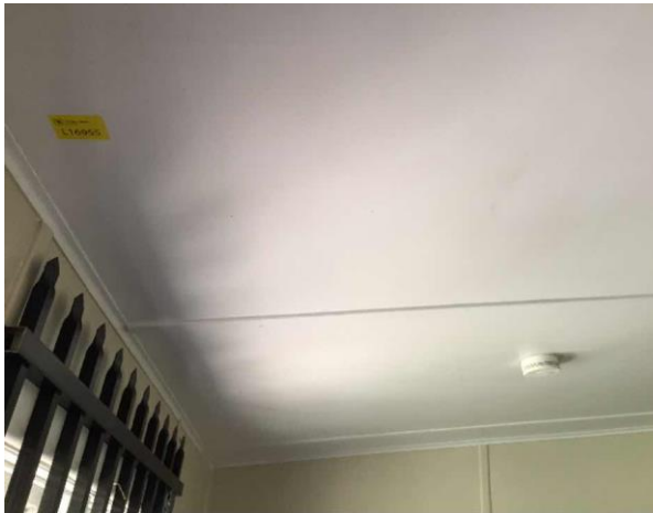
Line ID 116: Internal, GF, Bush Craft Building, Ceilings and Window Frames, White Paint - Lead Detected (5.8% w/w)
