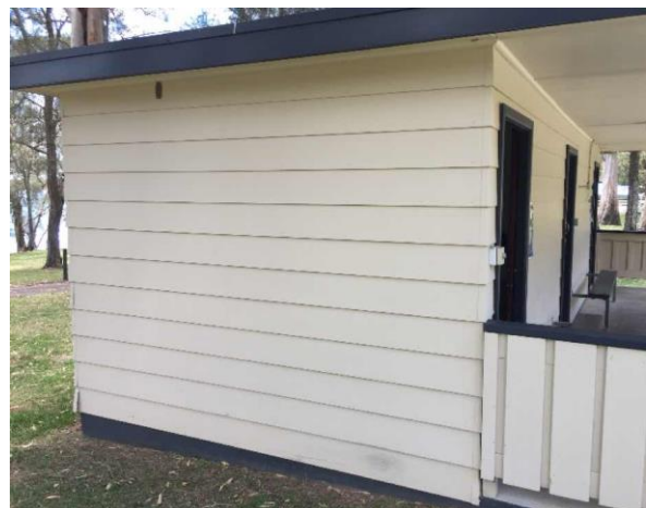
Line ID 113: External, GF, Tennis Court Amenities Block (North), Walls Throughout, Beige Paint - Lead Detected (<0.005% w/w)
