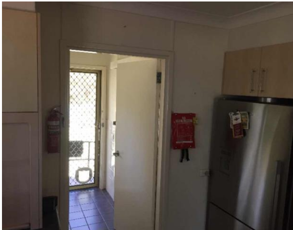
Line ID 86: Internal, GF, Residence 3 and Garage, Kitchen Walls, Fibre Cement Sheeting - Chrysotile, Amosite and Crocidolite Asbestos Detected
