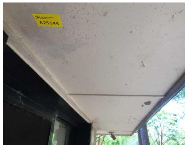
Line ID 42: External, GF, Residence 3 and Garage, House and Garage, Eaves, Fibre Cement Sheetting - Chrysotile Asbestos Detected
