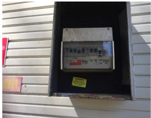
Line ID 16: External, GF, Conference Lodge, Southern Wall With Electrical Box, Bituminous Backing Board - Chrysotile Asbestos Detected
