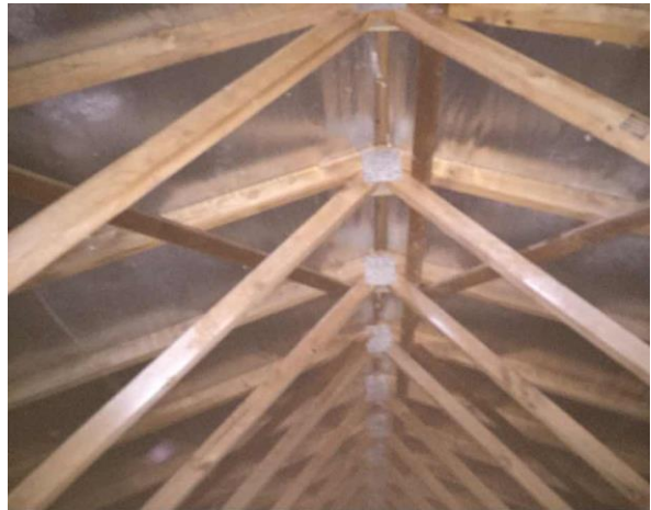
Line ID 146: Internal, GF, Residence 1 (Waratah House & Garage), House, Underside of Roof, Sarking Insulation - Suspected SMF
