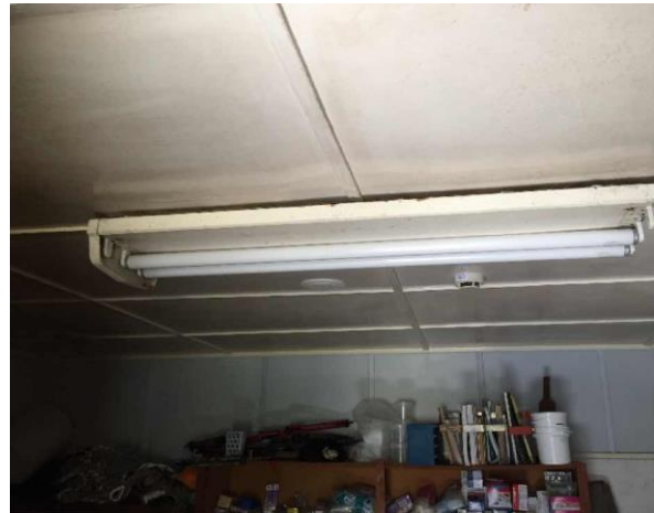
Line ID 152: Internal, GF, Equipment Store Building, Fluorescent Lights, Capacitor(s) - PCB Capacitor
