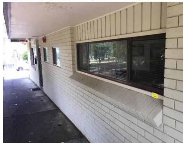
Line ID 93: External, GF, Administration/Office Building, Walls Throughout, Beige Paint - Lead Detected (<0.005% w/w)
