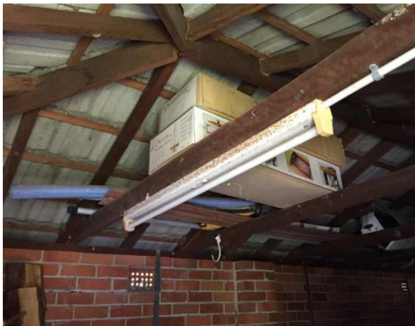
Line ID 153: Internal, GF, Residence 3 and Garage, Within Garage, Fluorescent Light, Capacitor(s) - Suspected PCB
