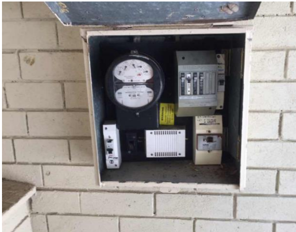
Line ID 37: External, GF, Residence 2, Electrical Box to South-eastern Corner, Bituminous Backing Board - Chrysotile Asbestos Detected
