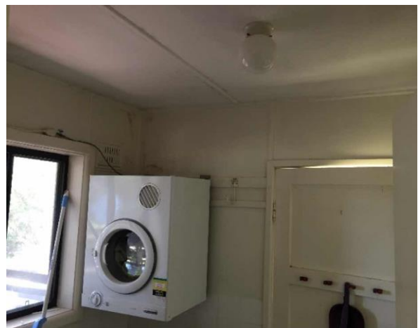
Line ID 89: Internal, GF, Residence 3 and Garage, Laundry Walls and Ceiling, Fibre Cement Sheeting - Chrysotile, Amosite and Crocidolite Asbestos Detected
