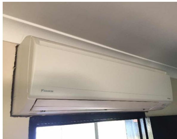
Line ID 166: Internal, GF, Banksia Lodge, Air Conditioning Units, R410A Hydrofluorocarbon (HFC) - Non ODS Refrigerant
