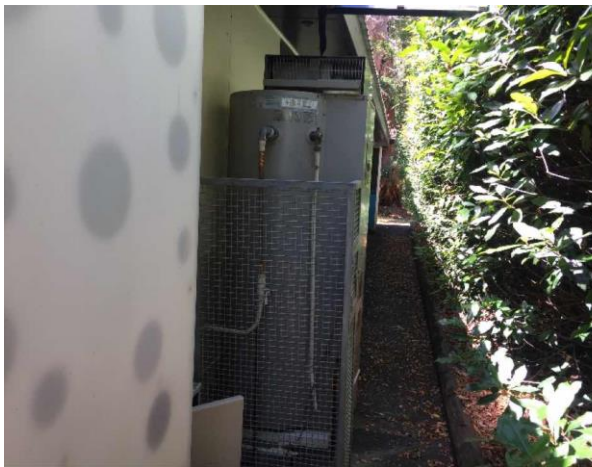
Line ID 124: External, GF, Casuarina Lodge, Western Wall, Hot Water Tank, Internal Insulation - Suspected SMF
