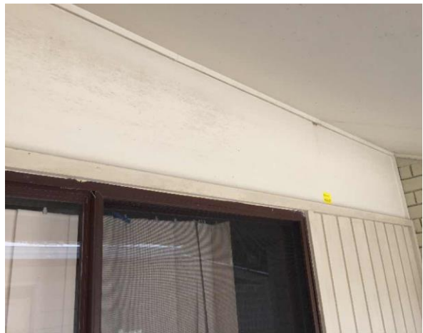
Line ID 36: External, GF, Residence 1 (Waratah House & Garage), Northern and Southern Elevations, Upper 1/4 Wall, Fibre Cement Sheeting - Chrysotile Asbestos Detected
