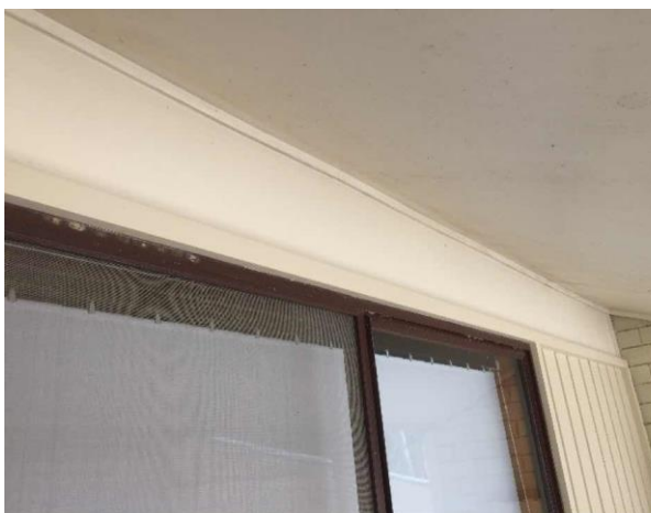
Line ID 41: External, GF, Residence, Northern and Southern Elevations, Upper 1/4 of Walls, Fibre Cement Sheetting - Chrysotile Asbestos Detected
