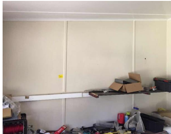
Line ID 117: Internal, GF, Bush Craft Building, Walls to Eastern Room, Beige Paint - Lead Detected (0.079% w/w)
