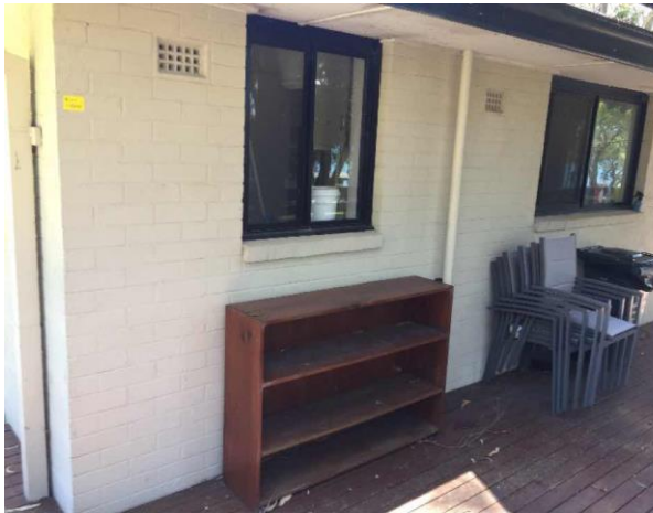
Line ID 110: External, GF, Residence 3 and Garage, Walls to House and Garage, Beige Paint - Lead Detected (0.008% w/w)
