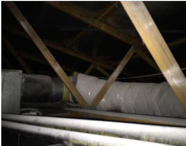
Line ID 134: Internal, GF, Administration/Office Building, Ceiling Space, Air Conditioning Ductwork, Insulation Material - Suspected SMF
