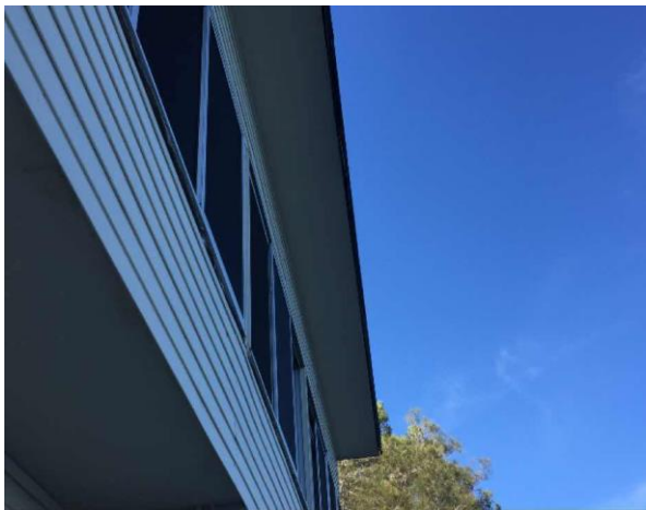
Line ID 29: External, GF, Recreational Hall, Eaves to Eastern and Western Elevations, Fibre Cement Sheetting - Chrysotile Asbestos Detected
