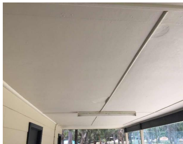
Line ID 48: External, GF, Tennis Court Amenities Block (North), Awning and Eaves (All Elevations), Fibre Cement Sheeting - Chrysotile Asbestos Detected
