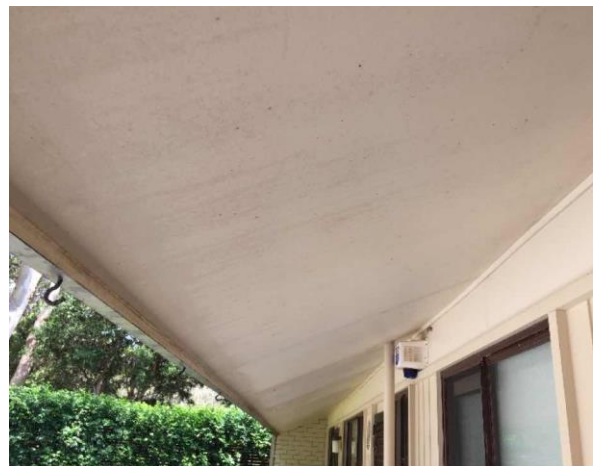
Line ID 40: External, GF, Residence 2 (Wattle House & Garage), House Northern and Southern Elevations, Porch Ceiling, Fibre Cement Sheetting - No Asbestos Detected
