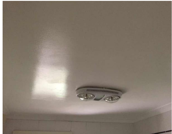
Line ID 85: Internal, GF, Residence 3 and Garage, Bathroom Ceiling, Fibre Cement Sheeting - Chrysotile, Amosite and Crocidolite Asbestos Detected
