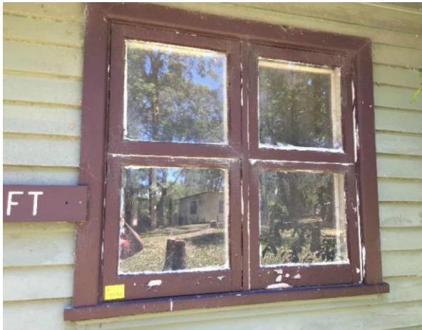
Line ID 96: External, GF, Bush Craft Building, Window and Door Frames, Brown (Dark) Paint - Lead Detected (0.19% w/w)
