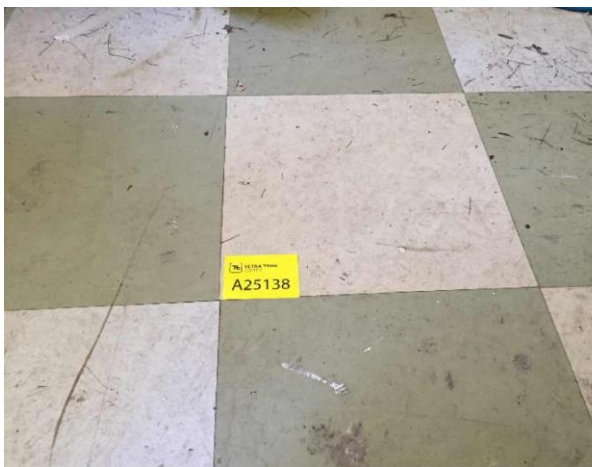
Line ID 65: Internal, GF, Bush Craft Building, Eastern Room, Cream Vinyl Floor Tiles - Chrysotile Asbestos Detected
