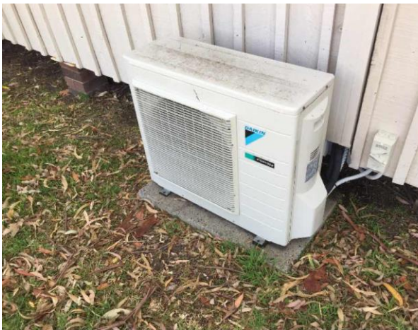
Line ID 161: External, GF, Holiday Units 1-8 (All Identical In Design), Air Conditioning Units, R410A Hydrofluorocarbon (HFC) - Non ODS Refrigerant
