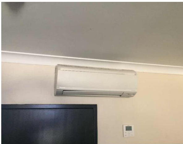
Line ID 165: Internal, GF, Acacia Lodge, Air Conditioning Units, R410A Hydrofluorocarbon (HFC) - Non ODS Refrigerant
