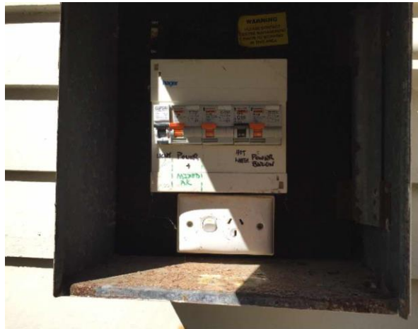
Line ID 22: External, GF, Gum Nut Lodge, Electrical Box to South Wall, Bituminous Backing Board - Chrysotile Asbestos Detected
