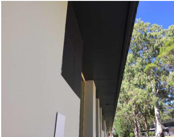
Line ID 1: External, GF, Acacia Lodge, Eaves Throughout, Fibre Cement Sheetting - No Asbestos Detected
