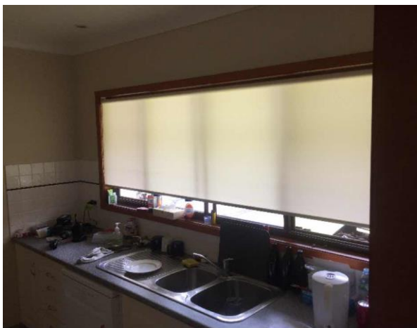
Line ID 82: Internal, GF, Residence 1 (Waratah House & Garage), South Wall of Kitchen, Fibre Cement Sheetting - Chrysotile Asbestos Detected
