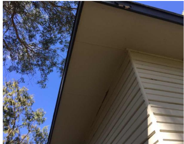
Line ID 14: External, GF, Conference Lodge, Eaves, Fibre Cement Sheetting - Chrysotile & Amosite Asbestos Detected
