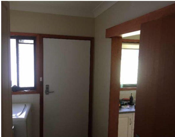
Line ID 81: Internal, GF, Residence 1 (Waratah House & Garage), Laundry, Toilet and Shower Walls, Fibre Cement Sheetting - Chrysotile Asbestos Detected
