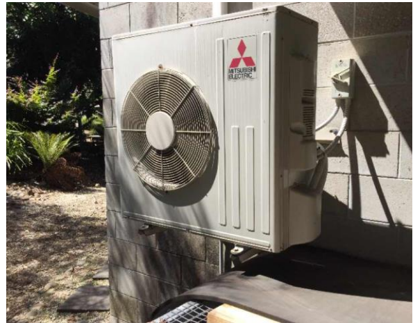
Line ID 158: External, GF, Dining Hall, Southern Elevation, Air Conditioning Unit, R410A Hydrofluorocarbon (HFC) - Non ODS Refrigerant
