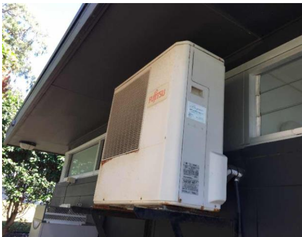
Line ID 155: External, GF, Bluegum Lodge, Southern Elevation, Air Conditioning Unit, R22 Hydrochlorofluorocarbon (HCFC) - ODS Refrigerant
