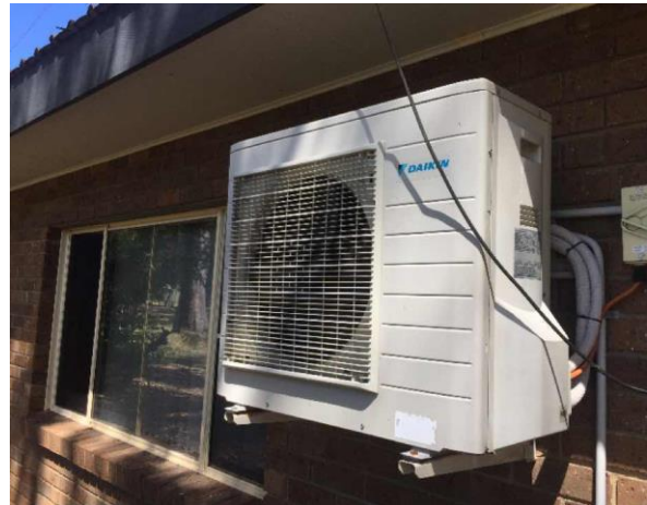
Line ID 164: External, GF, Staff Residence, Northern Wall, Air Conditioning Unit, R410A Hydrofluorocarbon (HFC) - Non ODS Refrigerant
