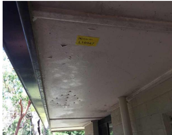
Line ID 109: External, GF, Residence 3 and Garage, Eaves to House and Garage, White Paint - Lead Detected (0.46% w/w)
