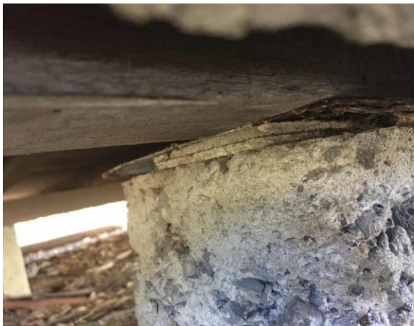
Line ID 23: External, GF, Gum Nut Lodge, Subfloor, Packers to Building Support Beams, Fibre Cement Sheet - Chrysotile Asbestos Detected
