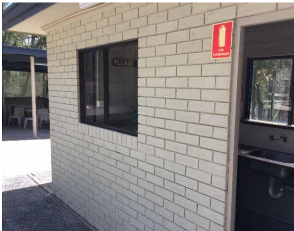
Line ID 104: External, GF, Holiday Units (1-8) Laundry, Walls, Grey Paint - Lead Detected (0.02% w/w)
