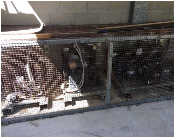
Line ID 157: External, GF, Dining Hall, Chiller Units, R404A Refrigerant - Non ODS Refrigerant
