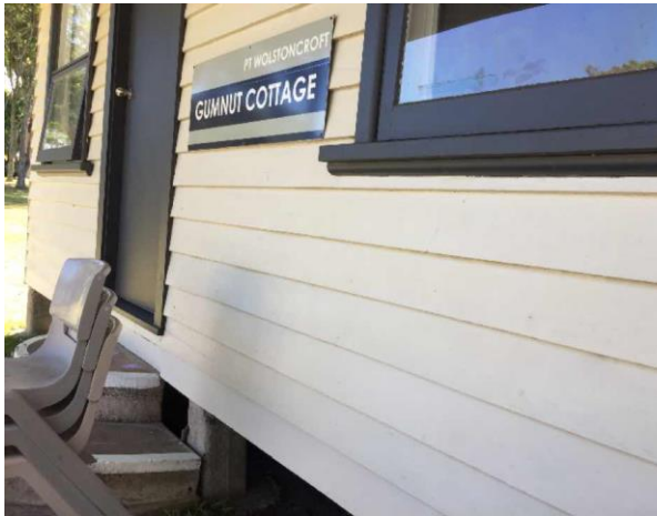
Line ID 102: External, GF, Gum Nut Lodge, Walls Throughout, Beige Paint - Lead Detected (7.1% w/w)
