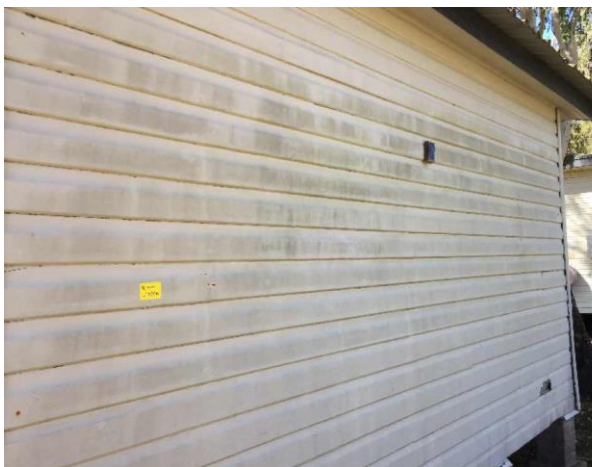
Line ID 100: External, GF, Equipment Store Building, Walls, Beige Paint - Lead Detected (7.1% w/w)
