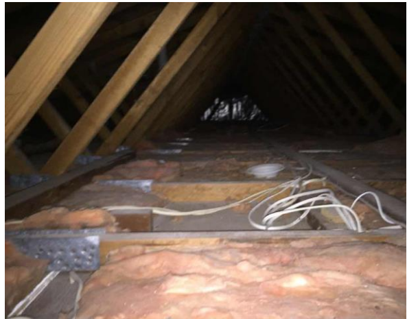
Line ID 148: Internal, GF, Residence 2 (Wattle House & Garage), House, Floor of Ceiling Void, Insulation Batts - Suspected SMF
