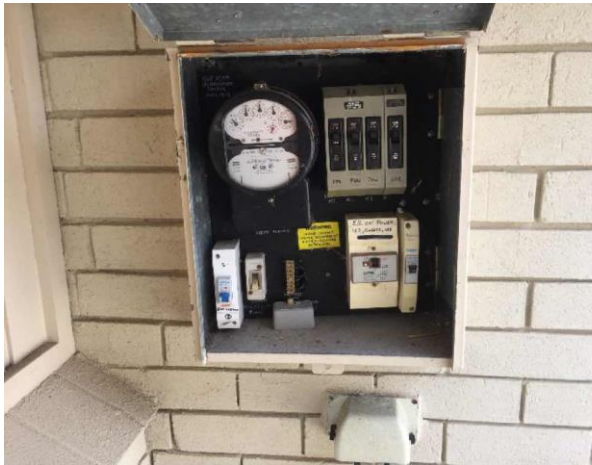
Line ID 31: External, GF, Residence 1, Electrical Box to South-eastern Corner, Bituminous Backing Board - Chrysotile Asbestos Detected
