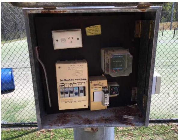
Line ID 45: External, GF, Ropes Course Store Building/Toilet, Light Pole Adjacent Tennis Court, Electrical Fuse Box , Bituminous Backing Board - Suspected Asbestos
