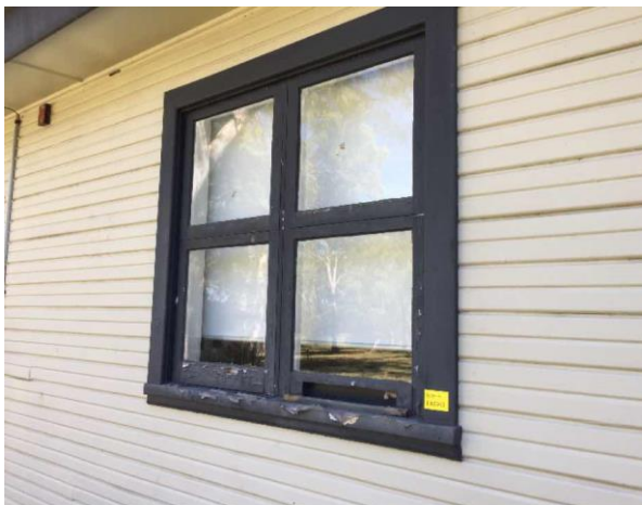
Line ID 98: External, GF, Conference Lodge, Windows and Trim Throughout, Grey (Dark) Paint - Lead Detected (1.9% w/w)
