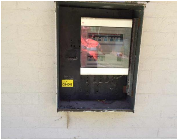
Line ID 43: External, GF, Residence 3 and Garage, Southern Elevation Within Fuse Box, Bituminous Backing Board - Chrysotile Asbestos Detected
