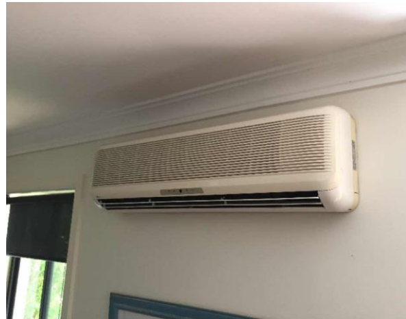
Line ID 170: Internal, GF, Residence 3 and Garage, Lounge Room, Air Conditioning Unit, R22 Hydrochlorofluorocarbon (HCFC) - ODS Refrigerant
