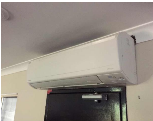
Line ID 167: Internal, GF, Casuarina Lodge, Air Conditioning Units, R410A Hydrofluorocarbon (HFC) - Non ODS Refrigerant
