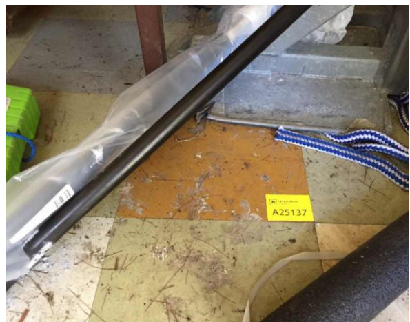
Line ID 66: Internal, GF, Bush Craft Building, Eastern Room, Orange Vinyl Floor Tiles - Chrysotile Asbestos Detected
