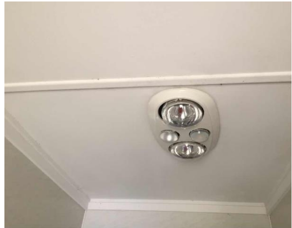
Line ID 87: Internal, GF, Residence 3 and Garage, Laundry Toilet Ceiling, Fibre Cement Sheeting - Chrysotile, Amosite and Crocidolite Asbestos Detected
