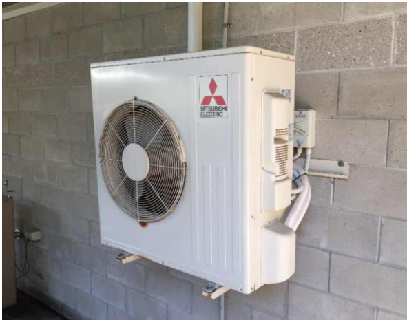
Line ID 159: External, GF, Dining Hall, Western Wall, Air Conditioning Unit, R410A Hydrofluorocarbon (HFC) - Non ODS Refrigerant
