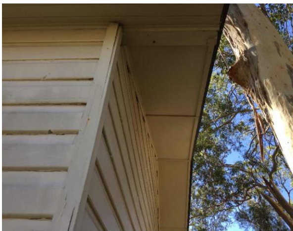
Line ID 17: External, GF, Equipment Store Building, Northern and Southern Elevations, Eaves, Fibre Cement Sheetting - Chrysotile & Amosite Asbestos Detected
