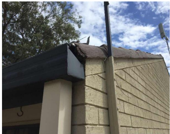
Line ID 30: External, GF, Residence 1 (Waratah House & Garage), Below Roof Tiles, Compressed Cement Sheetting - Chrysotile Asbestos Detected
