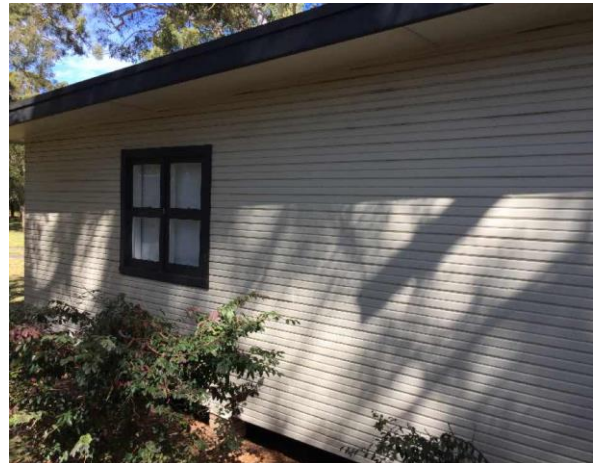
Line ID 97: External, GF, Conference Lodge, Walls, Beige Paint - Lead Detected (<0.005% w/w)
