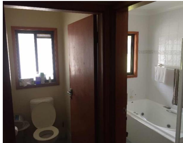
Line ID 81.1: Internal, GF, Residence 1 (Waratah House & Garage), Laundry, Toilet and Shower Walls, Fibre Cement Sheetting - Chrysotile Asbestos Detected
