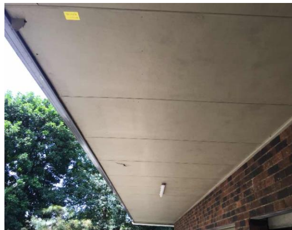
Line ID 52: External, GF, Workshop (Including Workshop Garage), Eaves Throughout, Fibre Cement Sheetting - No Asbestos Detected
