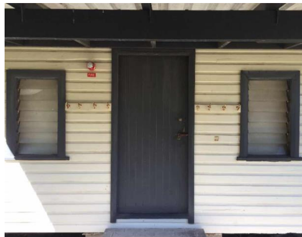
Line ID 99: External, GF, Equipment Store Building, Door, Window Frames and Trim, Grey (Dark) Paint - Lead Detected (1.9% w/w)
