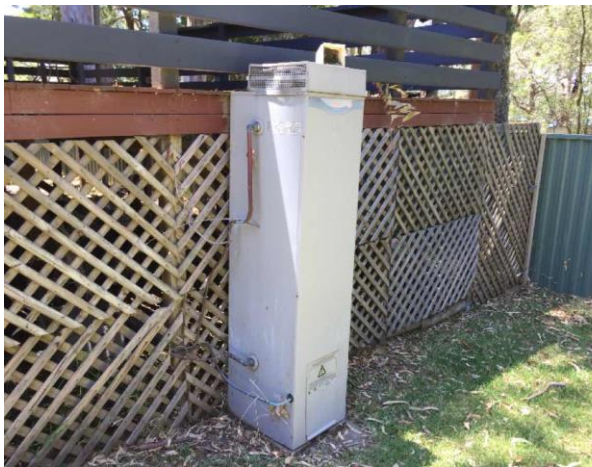
Line ID 130: External, GF, Residence 3 and Garage, South-eastern Corner, Hot Water Tank, Internal Insulation - Suspected SMF
