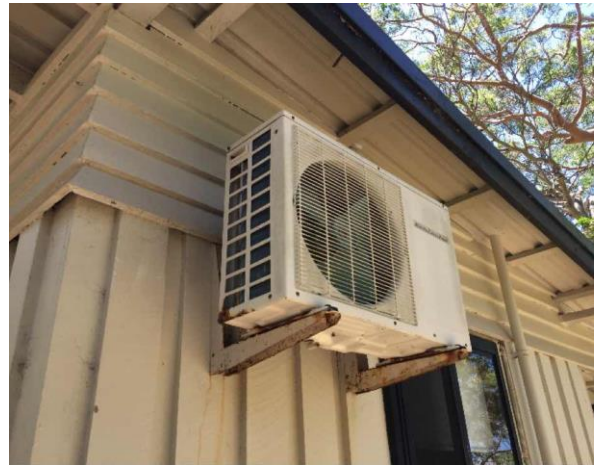
Line ID 160: External, GF, Hakea Lodges 1-3, Air Conditioning Units, R22 Hydrochlorofluorocarbon (HCFC) - ODS Refrigerant
