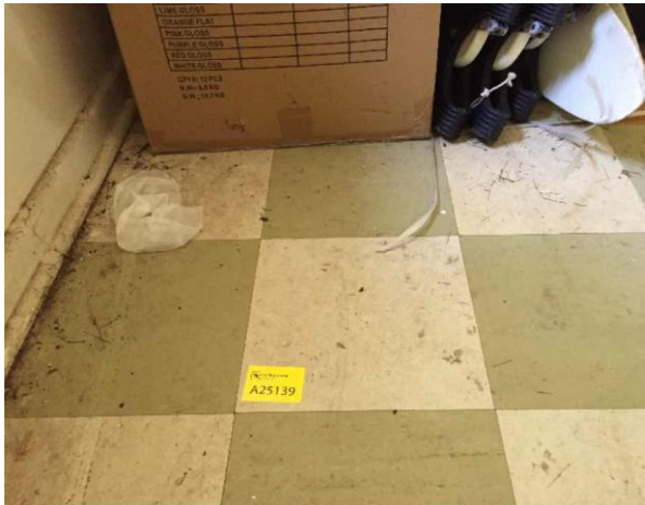
Line ID 67: Internal, GF, Bush Craft Building, Eastern Room, Light Grey Vinyl Floor Tiles - Chrysotile Asbestos Detected
