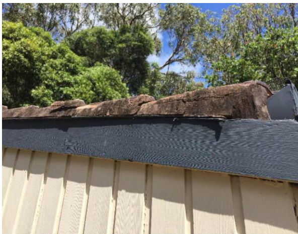
Line ID 39: External, GF, Residence 2 (Wattle House & Garage), House and Garage, Under Roof Tiles, Compressed Cement Sheetting - Chrysotile Asbestos Detected
