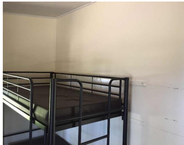
Line ID 119: Internal, GF, Hakea Lodges 1-3, Walls Throughout, Beige Paint - Lead Detected (0.006% w/w)
