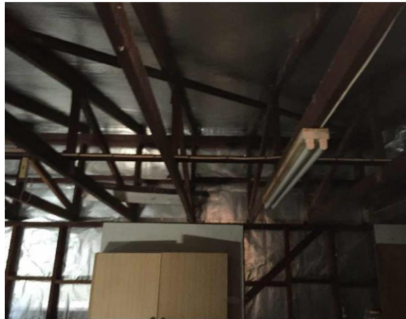
Line ID 129: External, GF, Residence 1 (Waratah House & Garage), Garage, Ceiling and Walls, Sarking Insulation - Suspected SMF
