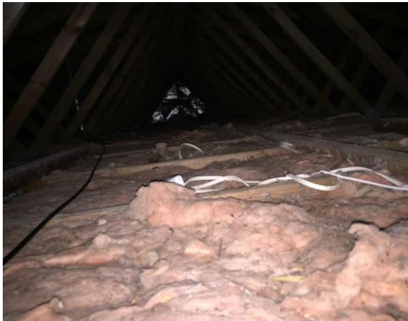
Line ID 145: Internal, GF, Residence 1 (Waratah House & Garage), House, Floor of Ceiling Void, Insulation Batts - Suspected SMF
