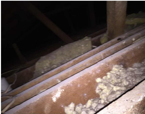
Line ID 151: Internal, GF, Residence 3 and Garage, Floor of Ceiling Void, Insulation Batts - Suspected SMF
