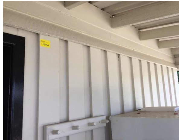
Line ID 103: External, GF, Hakea Lodges 1-3, Walls Throughout, Beige Paint - Lead Detected (<0.005% w/w)
