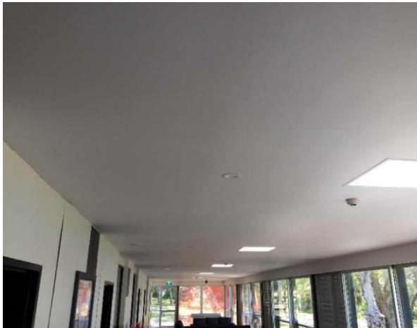
Line ID 73: Internal, GF, Grevillea Lodge, Veranda Ceiling, Fibre Cement Sheeting - No Asbestos Detected
