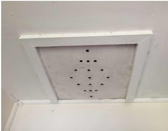
Line ID 90: Internal, GF, Residence 3 and Garage, Manhole Cover Within Laundry, Fibre Cement Sheetting - Chrysotile Asbestos Detected
