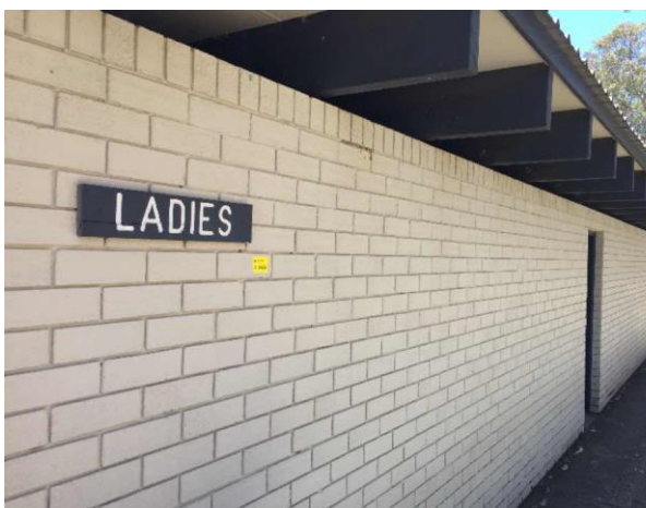
Line ID 106: External, GF, Pool House, Pool Store & Toilet Block, Walls Throughout, Beige Paint - Lead Detected (<0.005% w/w)
