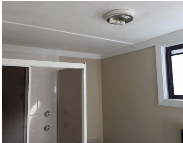
Line ID 74: Internal, GF, Gum Nut Lodge, Bathroom Walls and Ceiling, Fibre Cement Sheeting - Chrysotile & Amosite Asbestos Detected
