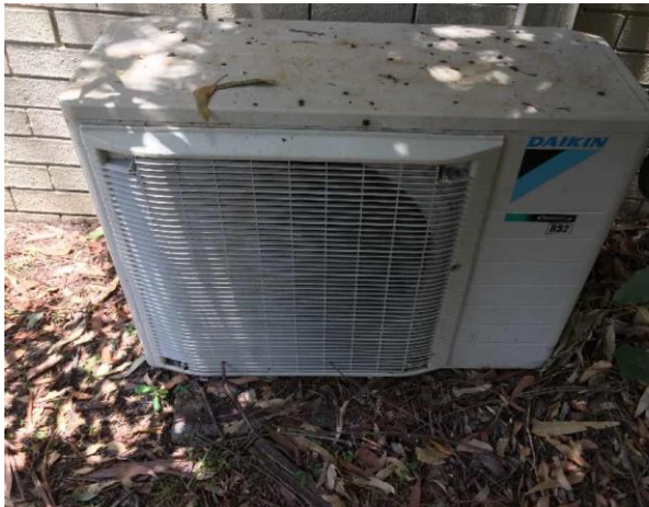
Line ID 163: External, GF, Residence 2 (Wattle House & Garage), Eastern Wall, Air Conditioning Unit, R32 Refrigerant - Non ODS Refrigerant
