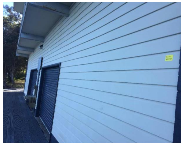
Line ID 54: External, Basement, The Boat Shed, Cladding to Western Wall, Compressed Cement Sheetting - Chrysotile Asbestos Detected
