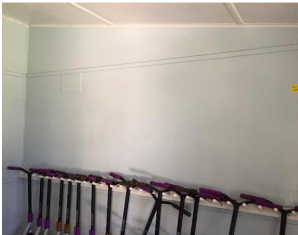
Line ID 118: Internal, GF, Bush Craft Building, Walls to Western Room, Blue Paint - Lead Detected (0.14% w/w)
