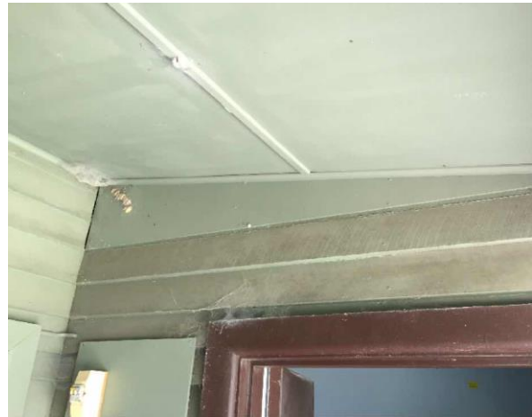
Line ID 10: External, GF, Bush Craft Building, Infill Panels to Upper Porch Walls, Fibre Cement Sheetting - Chrysotile & Amosite Asbestos Detected
